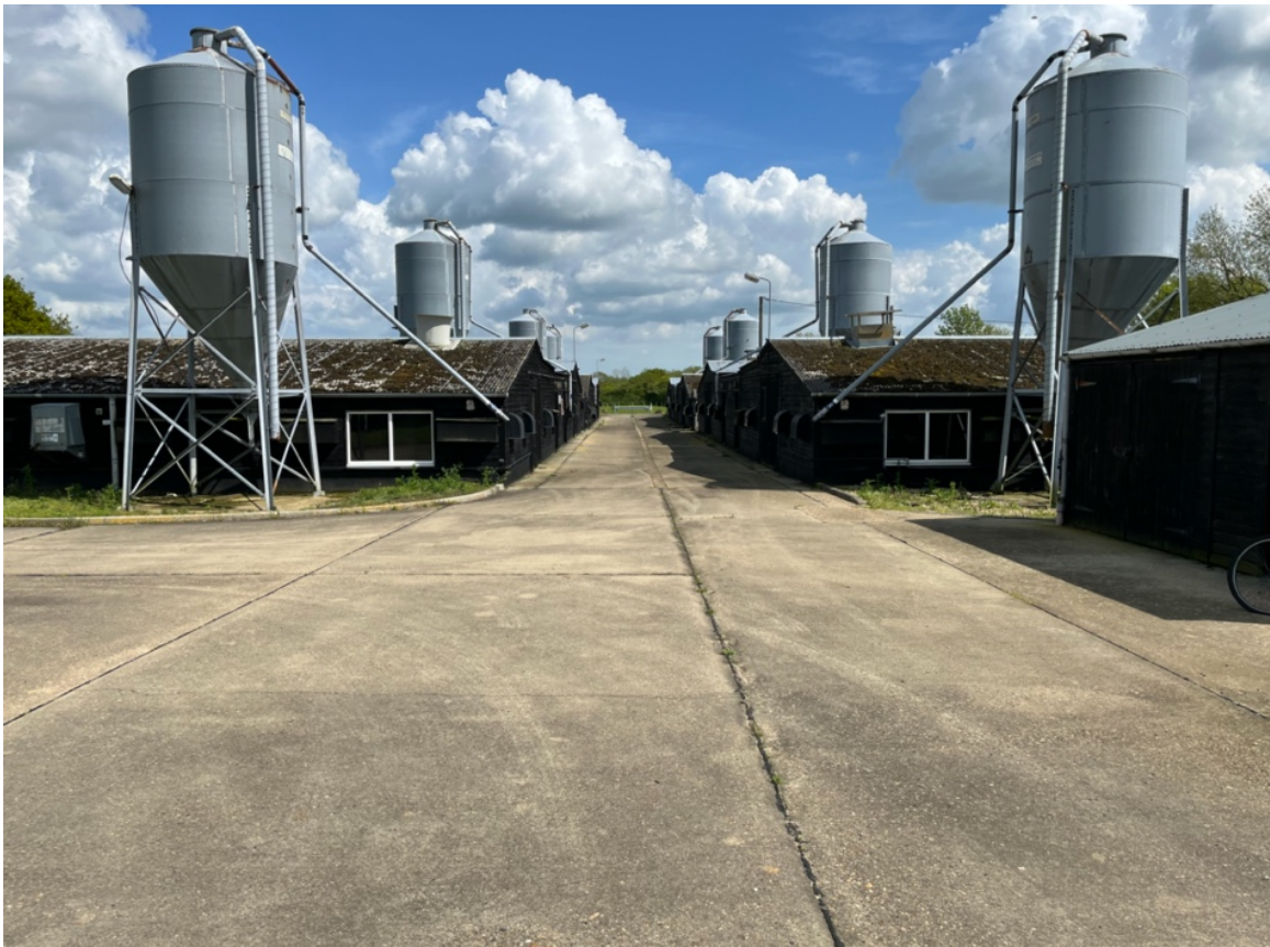
Photo 1 – View of the buildings/tanks to be demolished (front 2no. poultry houses being retained).
