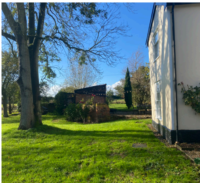
View towards existing wall and outbuildings from the east
