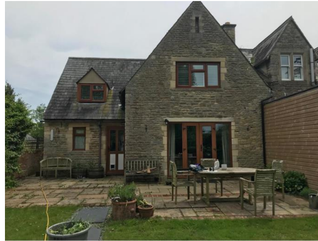
North (rear) elevation. Large neighbouring wooden structure can be seen to the right of the photo.
