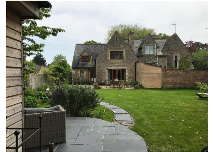
North (rear) elevation. Large neighbouring wooden structure can be seen to the right of the photo.
