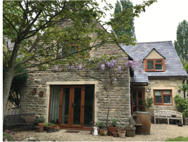
South elevation. Demonstrating current window casements and offset front door.
