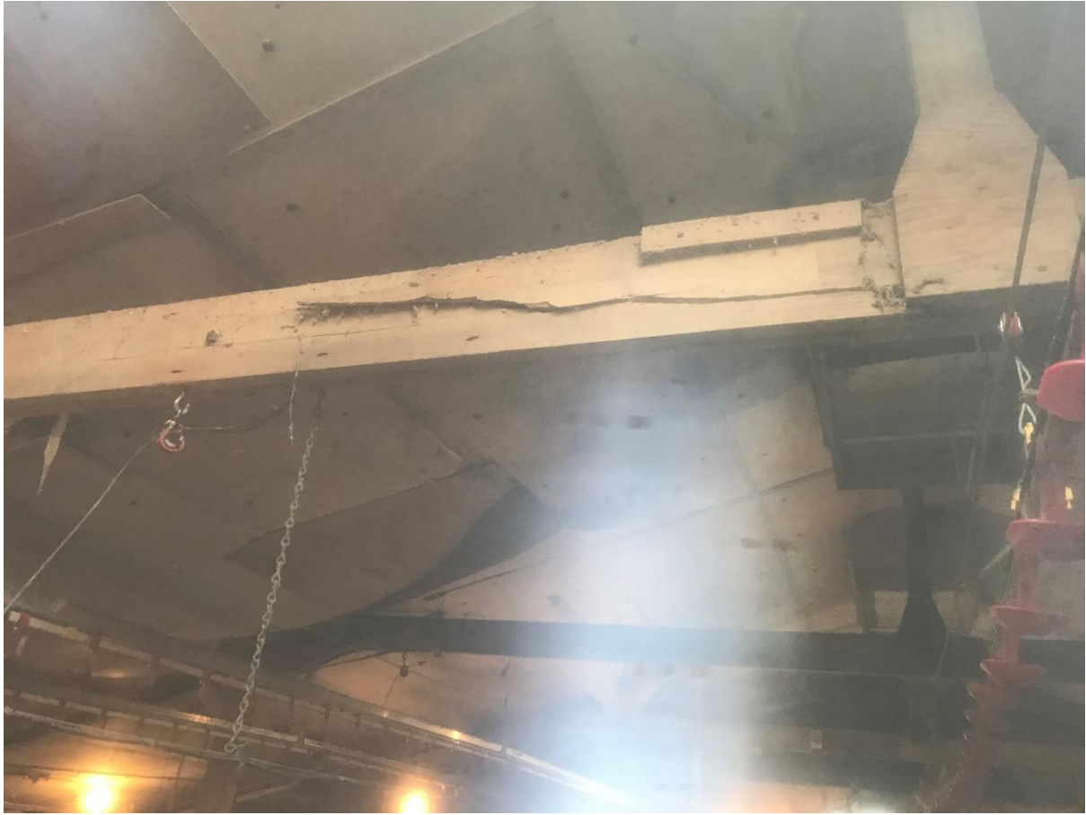
Photograph 9 – Split to Roof Tie
