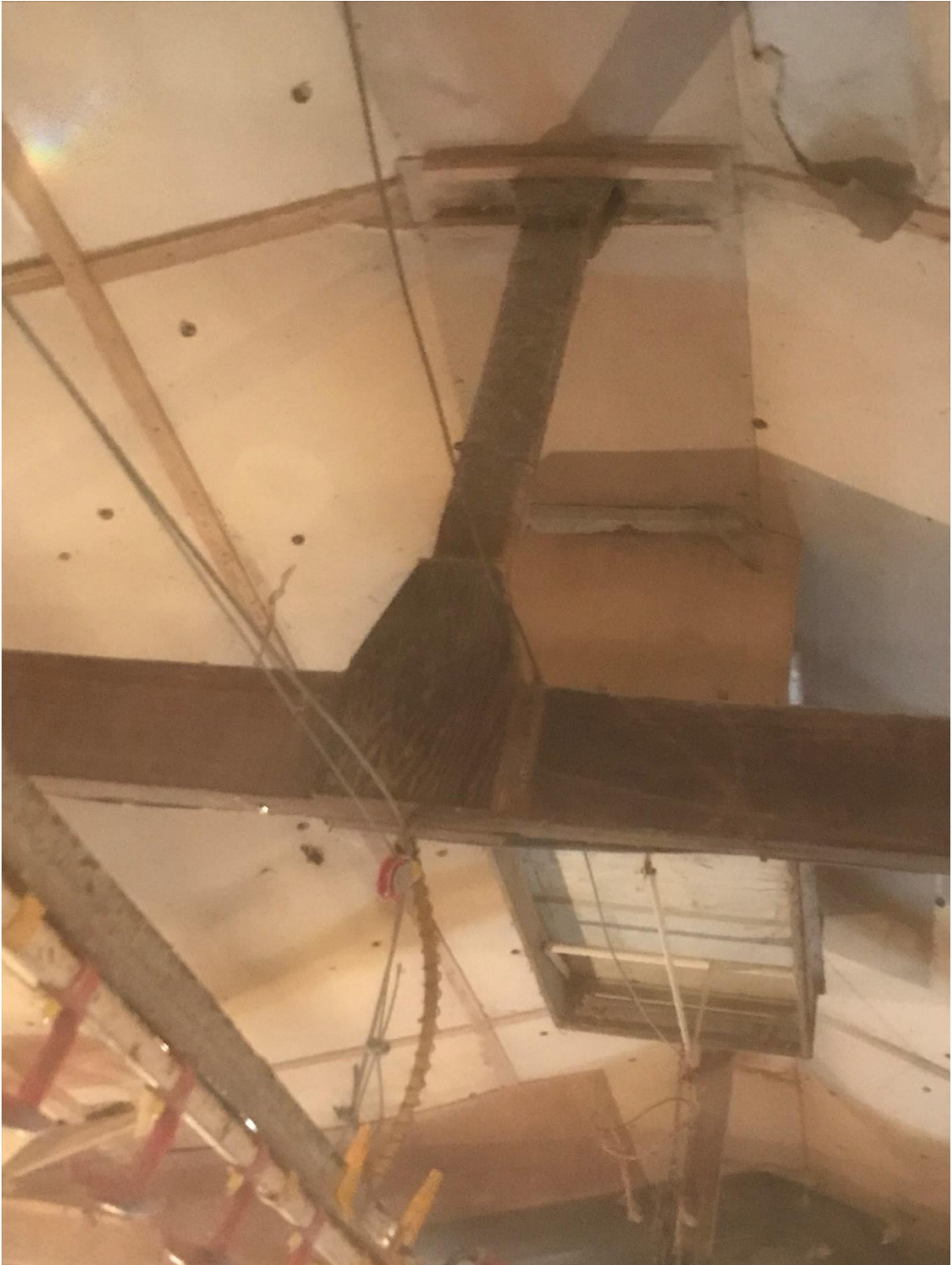
Photograph 8 - Typical Ply Gusset Connections to Roof "Truss"
