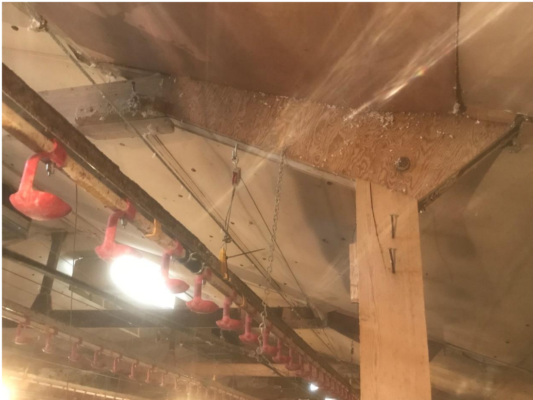
Photograph 6 – General View of “Key” Joint Detail Post to Rafter
