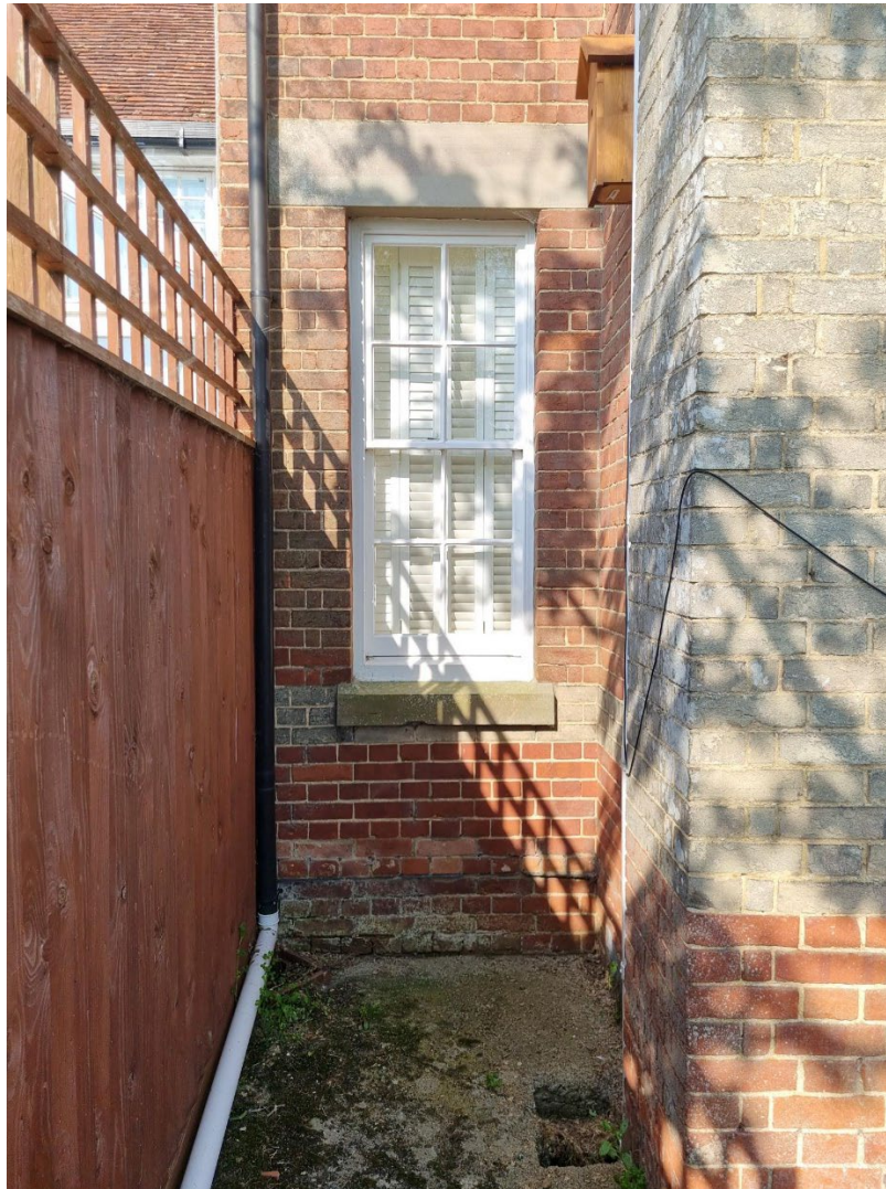
Figure 1. Existing sash window.
