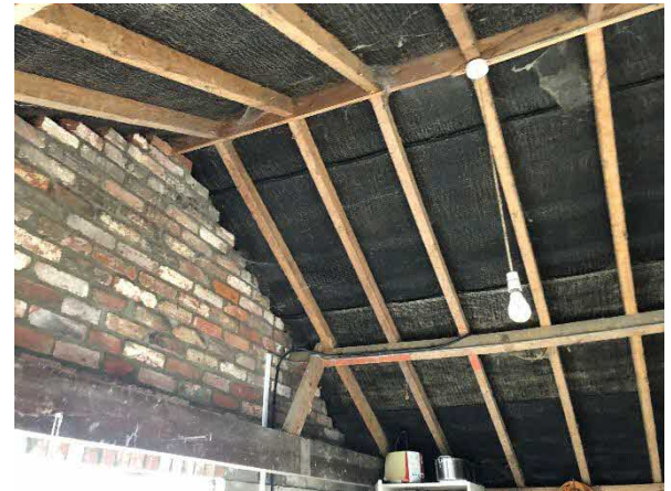
Photo 6: Internal view of Building 1
