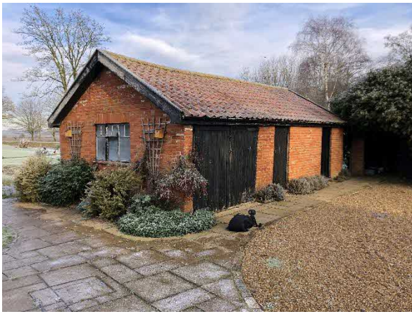
Photo 3: Building 1, south western facades
