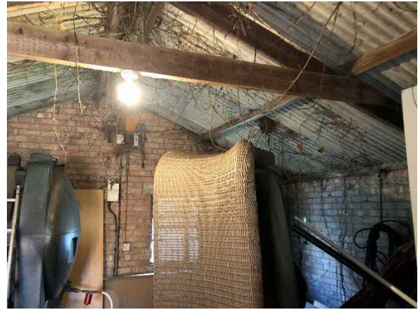
Photo 10: Internal view of Building 2
