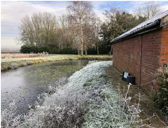
Photo 5: Bank of moat immediately to north Building 1
