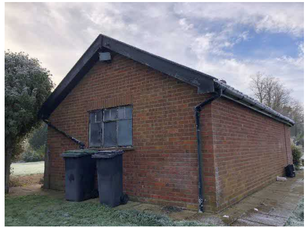
Photo 4: Building 1, north eastern facades
