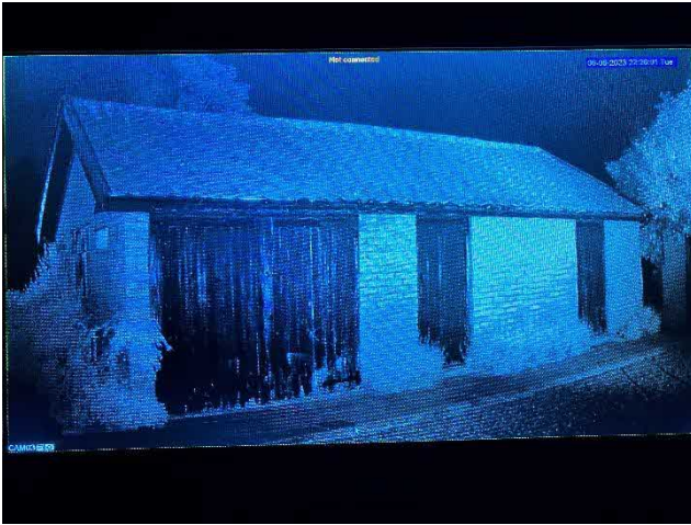
Photo 11: SANNCE IR camera view of south western façade of Building 1
