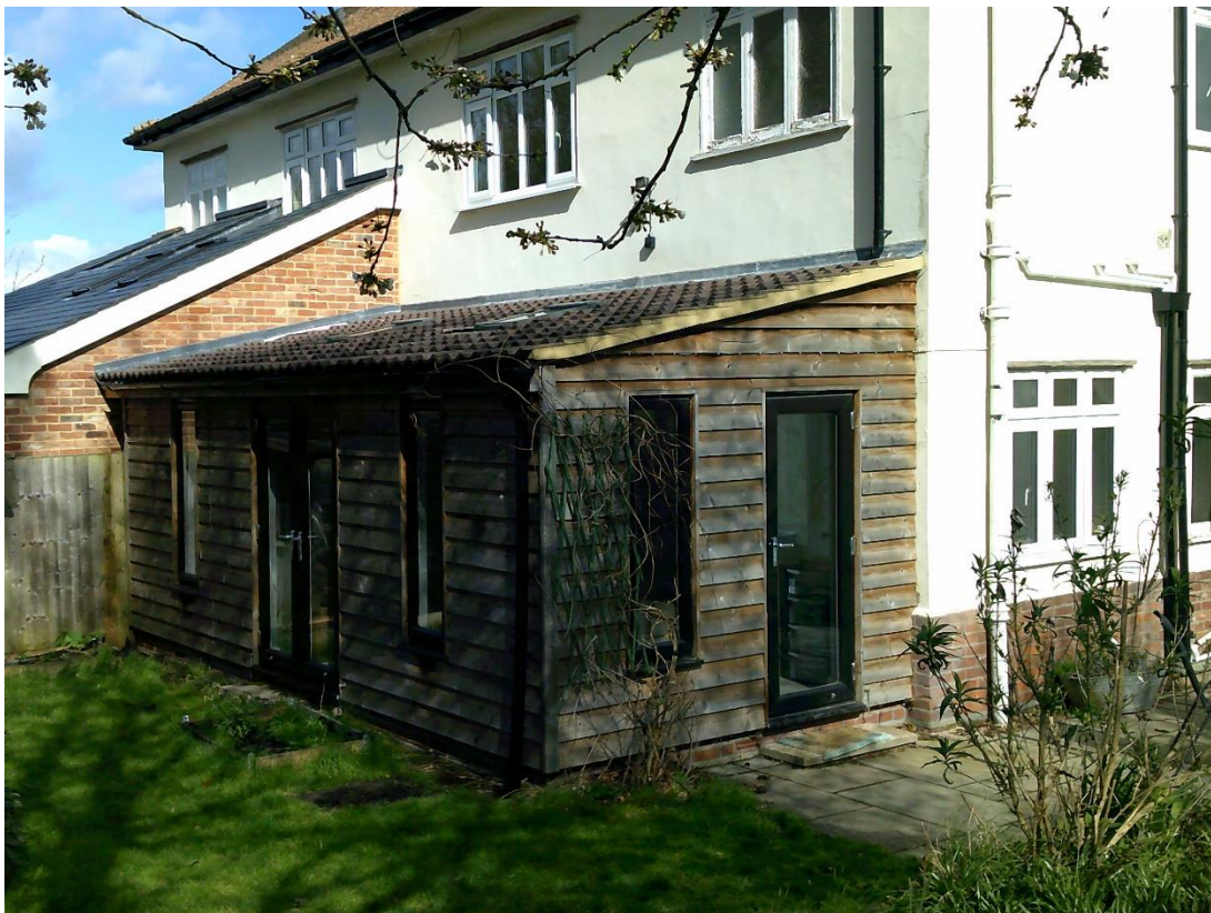
Existing rear extension
