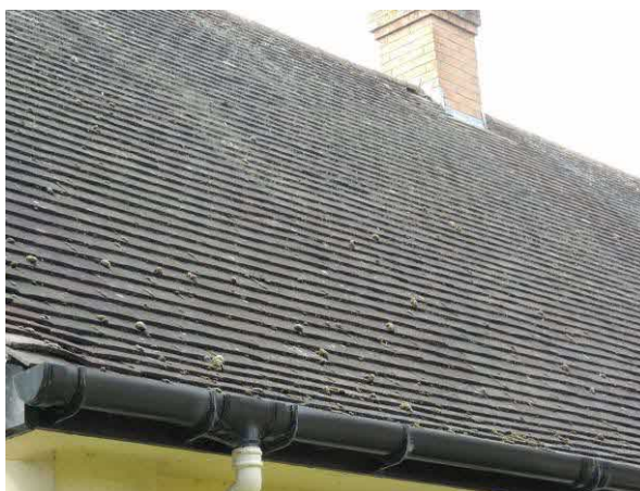
Note tight seal to roof tiles
