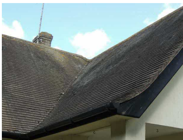
Note tight seal to roof tiles
