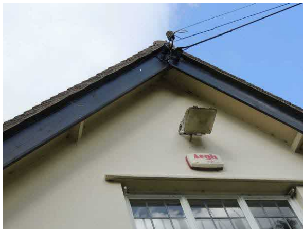
Note tight seal to gable
