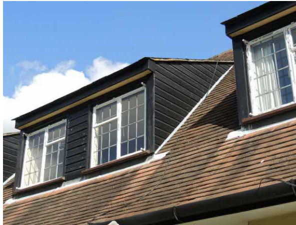
Note tight seal to tongue and groove cladding
