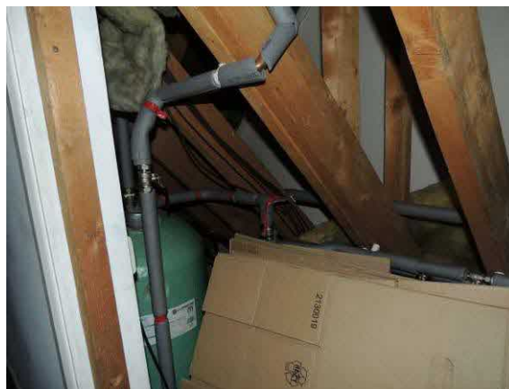
Note lack of evidence of bats in eaves cupboard
