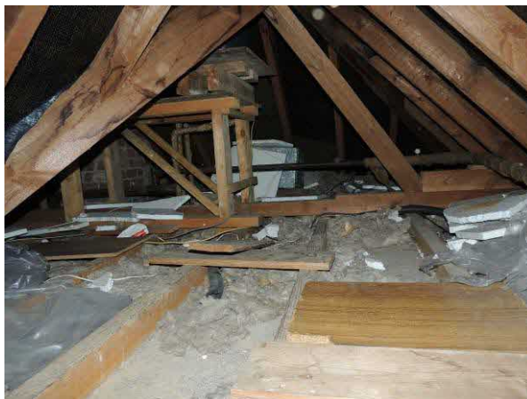
Note lack of evidence of bats on floor of loft
