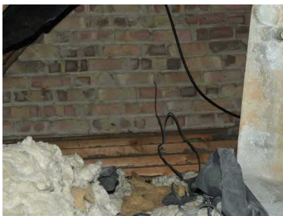
Note lack of evidence of bats on floor of loft
