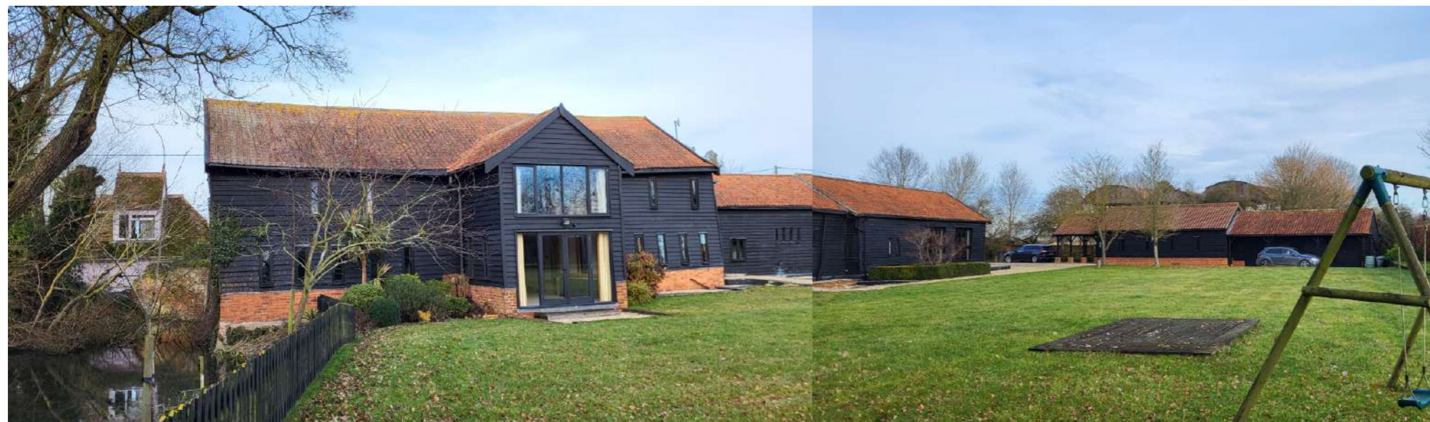
3- Image looking north at original barn, annexe and later detached out-buildings
