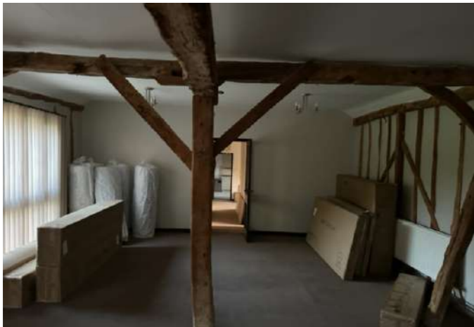
9- Existing timber beams and posts within annexe to be retained and expressed within remodelled master bedroom suite.
