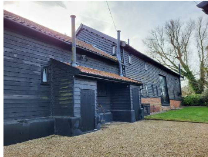
Image 1 - Lean-to boiler cupboards to be demolished
