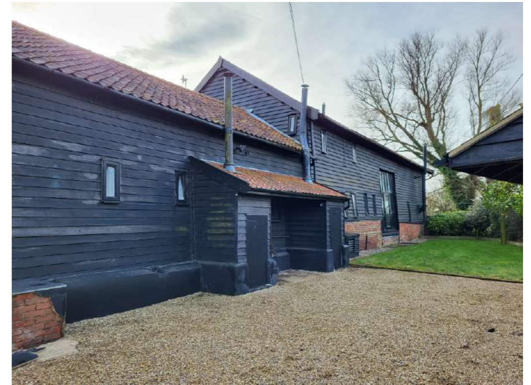
2- Image looking south-west at north-west facing elevation
