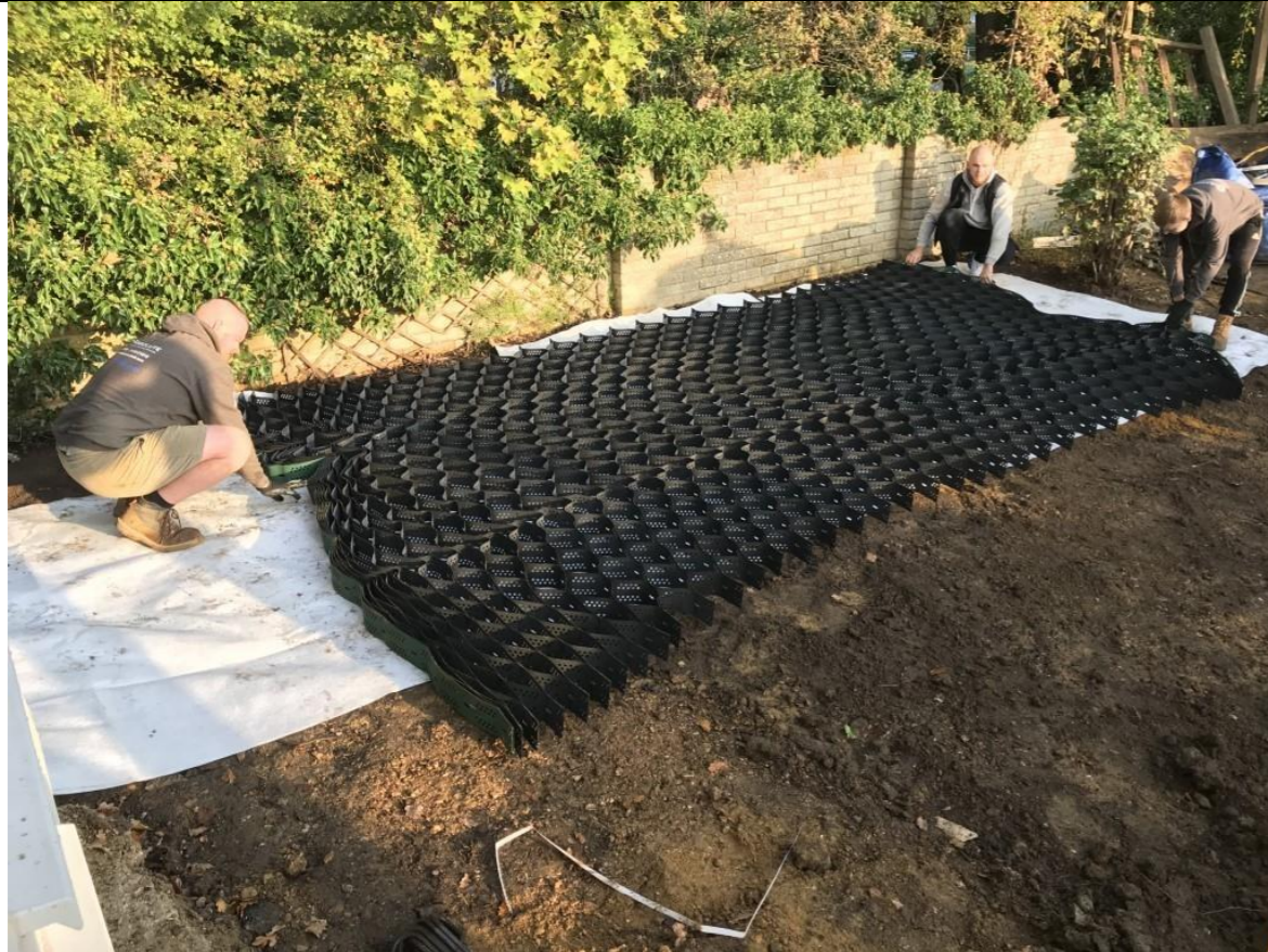
Fill with non-fines aggregate
