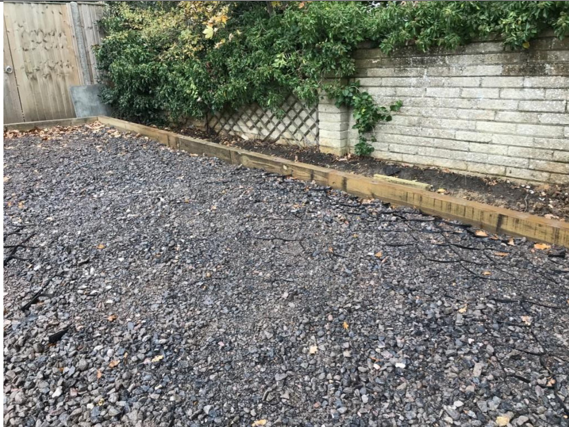
Fill with non-fines aggregate
