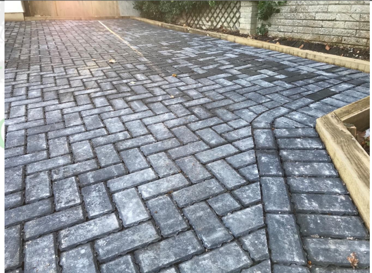
Lay permeable block paving on cellular confinement.
