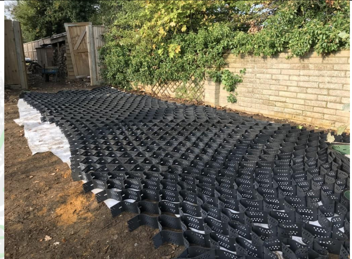
Lay permeable block paving on cellular confinement.
