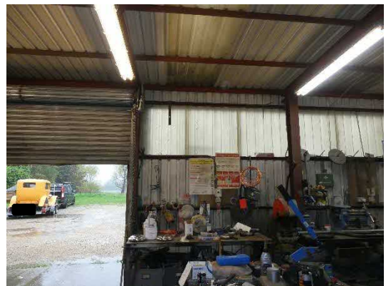
Photograph 6: Interior view of the lean-to extension
