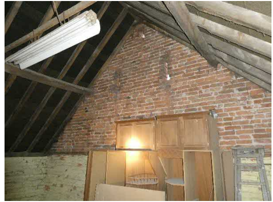
Photograph 2: Interior view of the first floor
