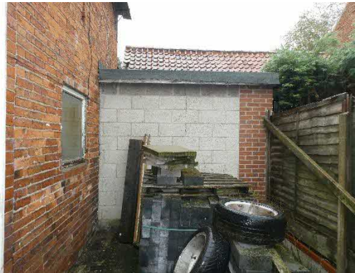
Photograph 8: Flat-roofed link extension on the eastern side
