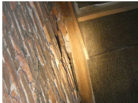
Photograph 18: Clean gap at the verge of the brick barn
