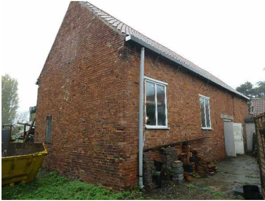
Photograph 1: Exterior view of the brick barn
