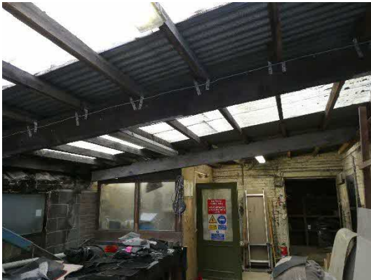
Photograph 7: Link extension between the brick barn and the outbuildings
