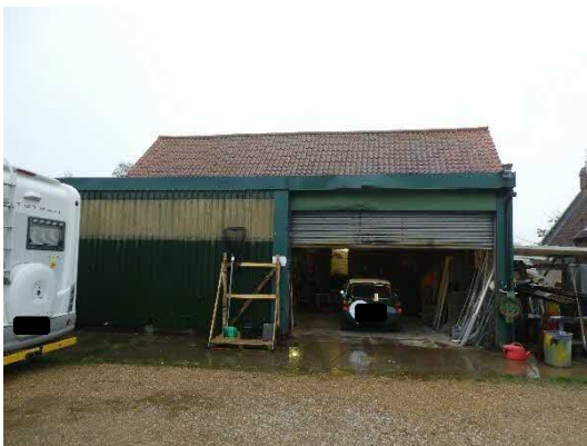
Photograph 5: Exterior view of the lean-to extension
