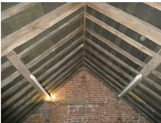
Photograph 3: View of the roof structure
