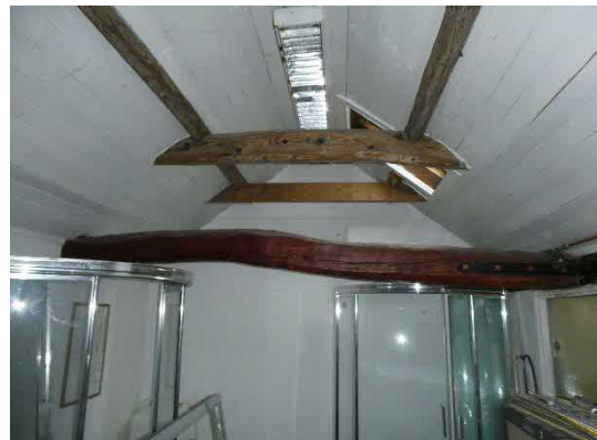
Photograph 10: Interior view of one of the westernmost outbuildings with the roof boarded out
