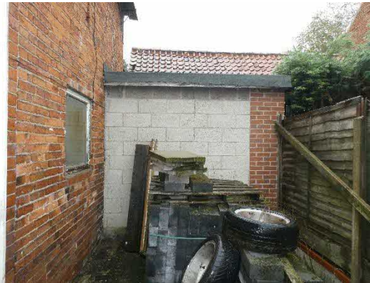
Photograph 8: Flat-roofed link extension on the eastern side
