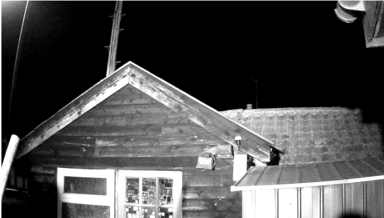
Photograph 1: Screenshot showing the field of view of the infrared camera, capturing the western elevation and roof structure of B1b. Taken at the darkest point of the survey.
