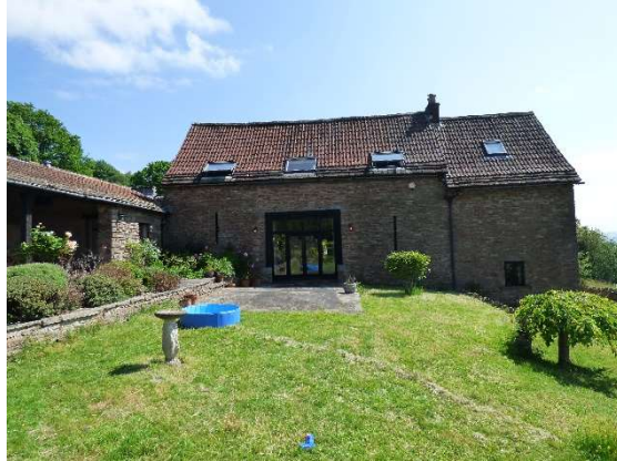
Photo 4: Converted barn and open-sided byre viewed from the west.
