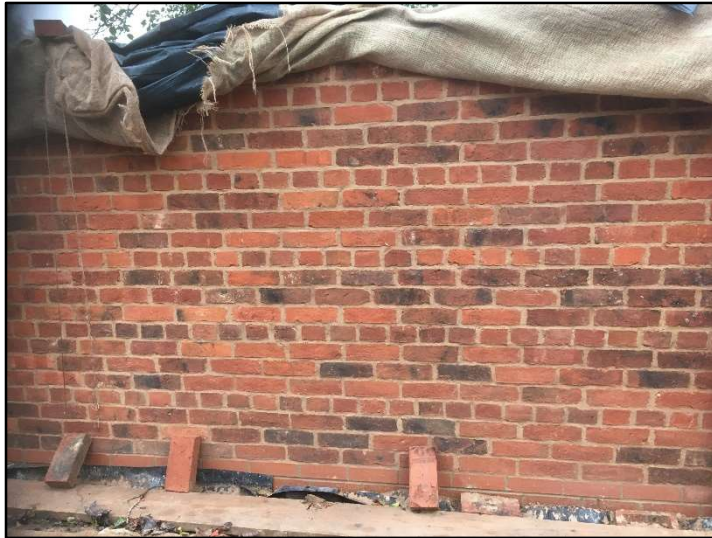
Figure 17 - New brick wall enclosing the western boundary of the application site (Hoar Cross handmade bricks).
