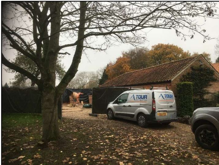
Figure 15 - Rear of the former stables.
