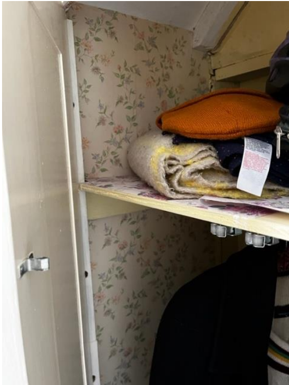
3 – The wall in the kitchen, the boxing will be removed (1980's) and a radiator fixed to the floor with pipes surface mounted.
