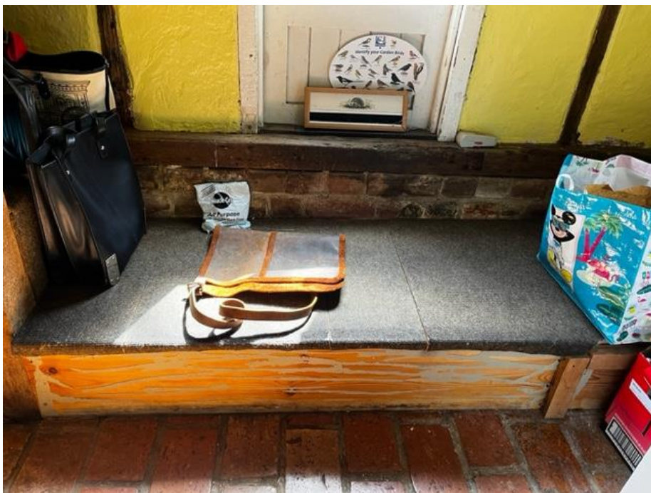
4 – Wall in the sitting room, radiator fixed to the floor with pipes surface mounted.
