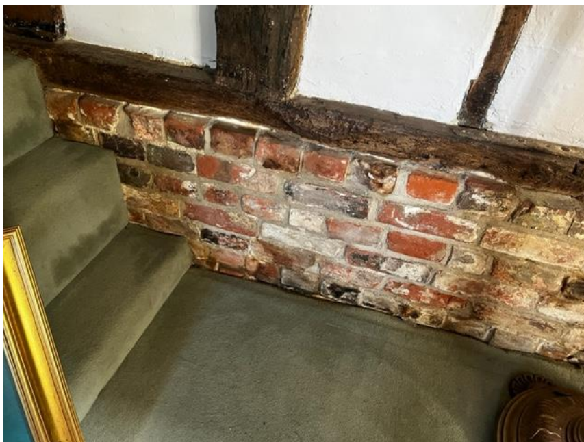
5 – Wall in the snug showing where pipes will be surface mounted.
