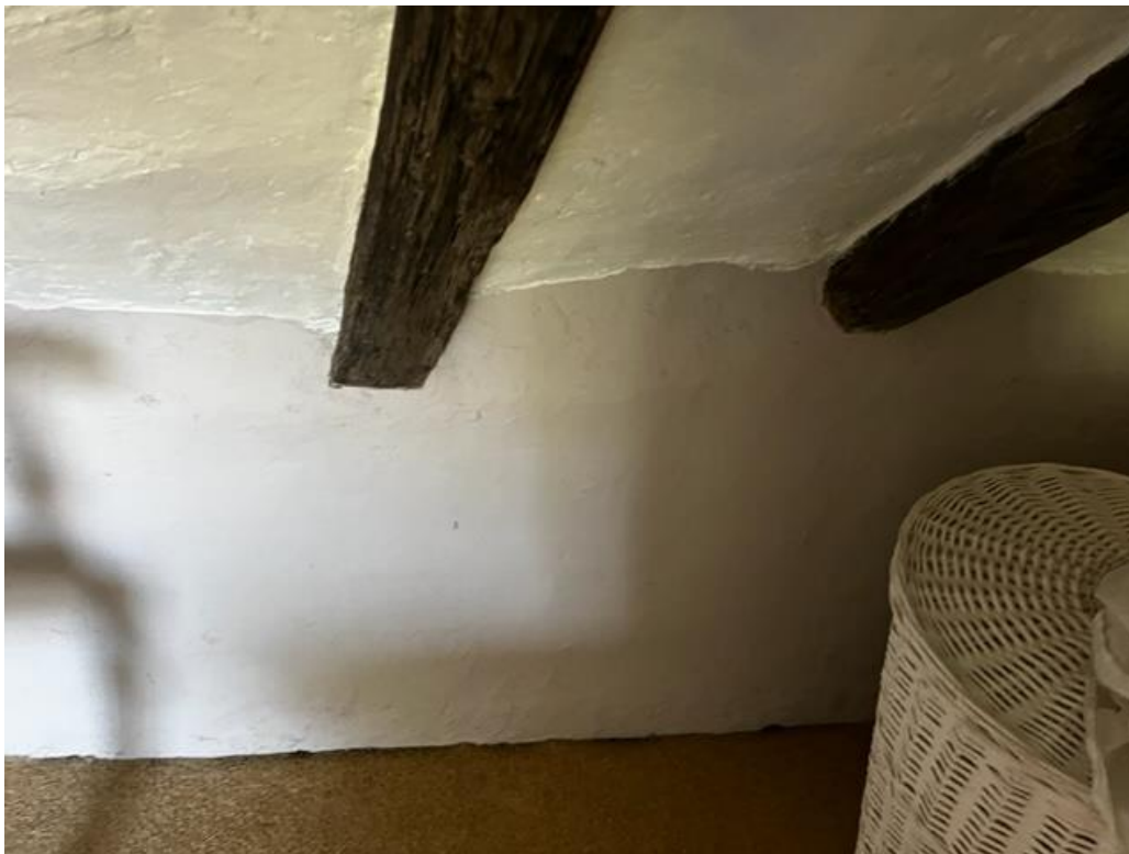
10 - Wall in bathroom which will have floor mounted towel rail
