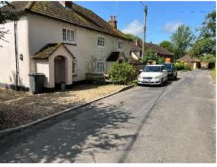
**Photo 3.** This photo shows the 8m curb length in detail which this planning application seeks to drop from 12cm to 2cm to generate off-street parking. The front garden outside Jasmine Cottage would then be graveled to mirror the off-street parking at the neighboring house, Honeysuckle Cottage.
