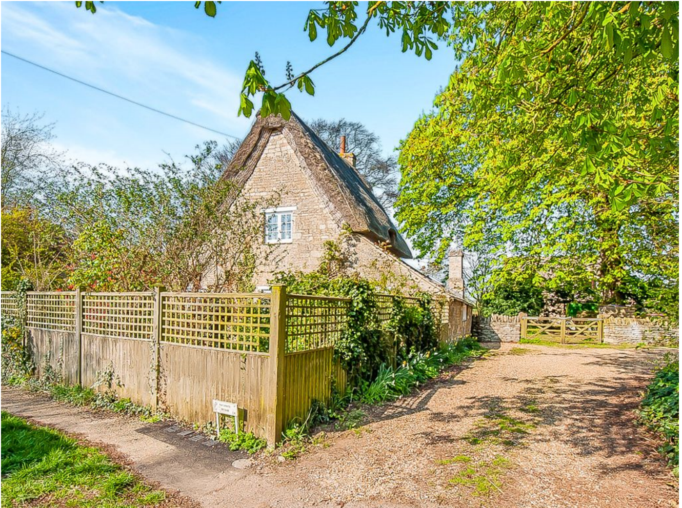
View of the old closeboarded and trellis topped timber fencing prior to replacement.
