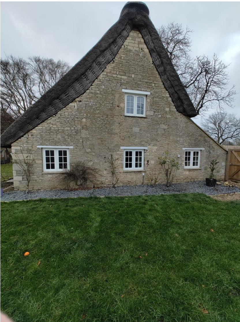
View of the front south west facing front elevation of the cottage as existing
