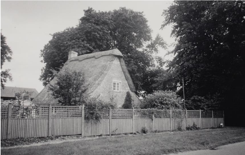
View of the old closeboarded and trellis topped timber fencing prior to replacement – no date.
