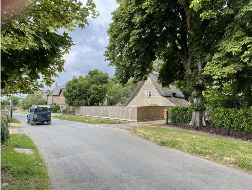
View of the existing vertical close boarded timber boundary fence abutting the road.
