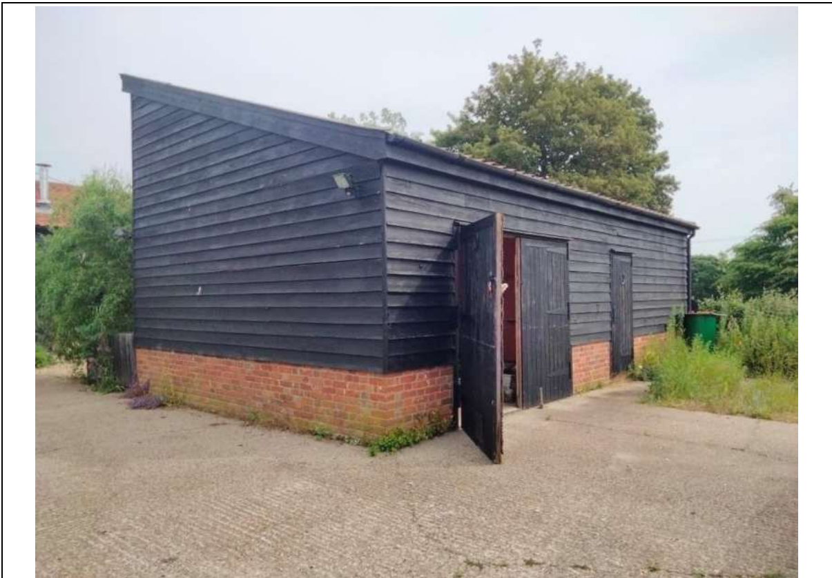
Photo 1 – Barn and hardstanding – Southern and Western Elevations
