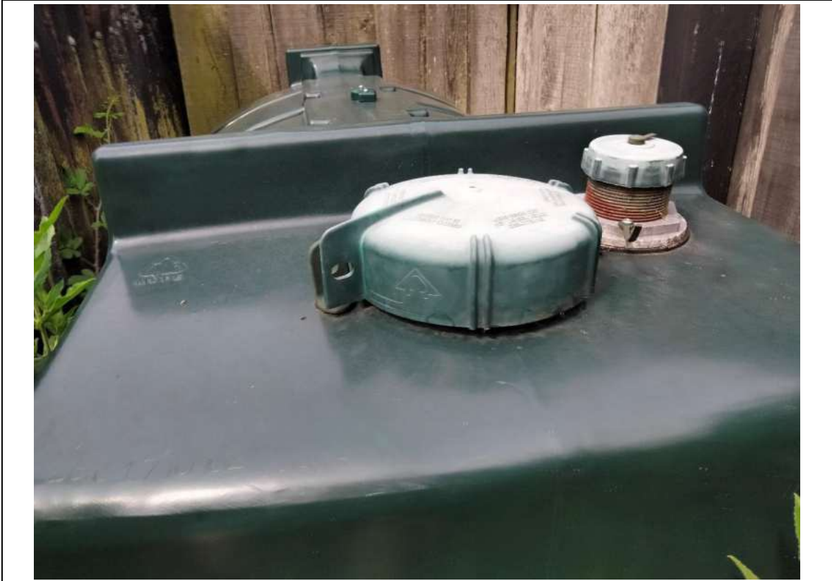
Photo 2 – Plastic internally banded heating oil tank
