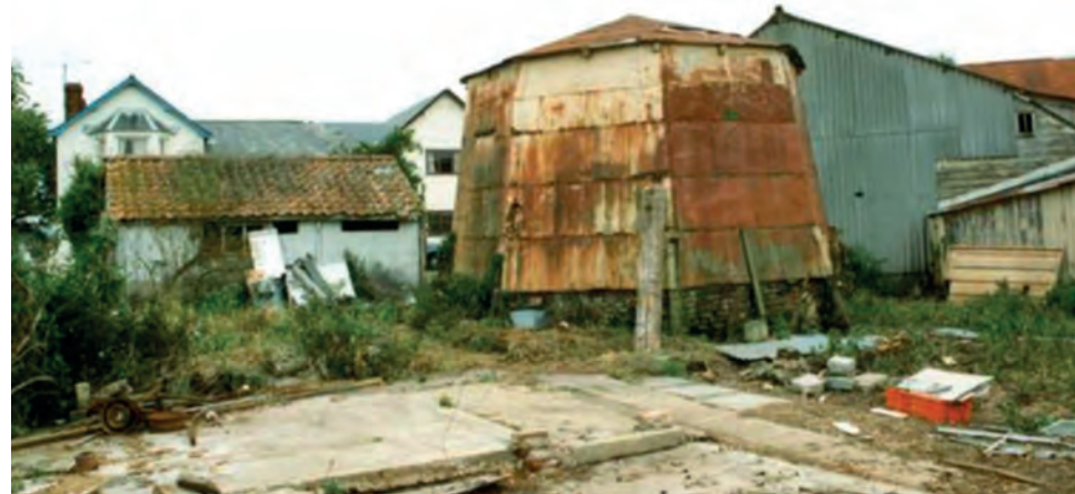
Above: Site photograph showing additional asbestos outbuildings. Right: Site location plan showing additional asbestos outbuildings.
