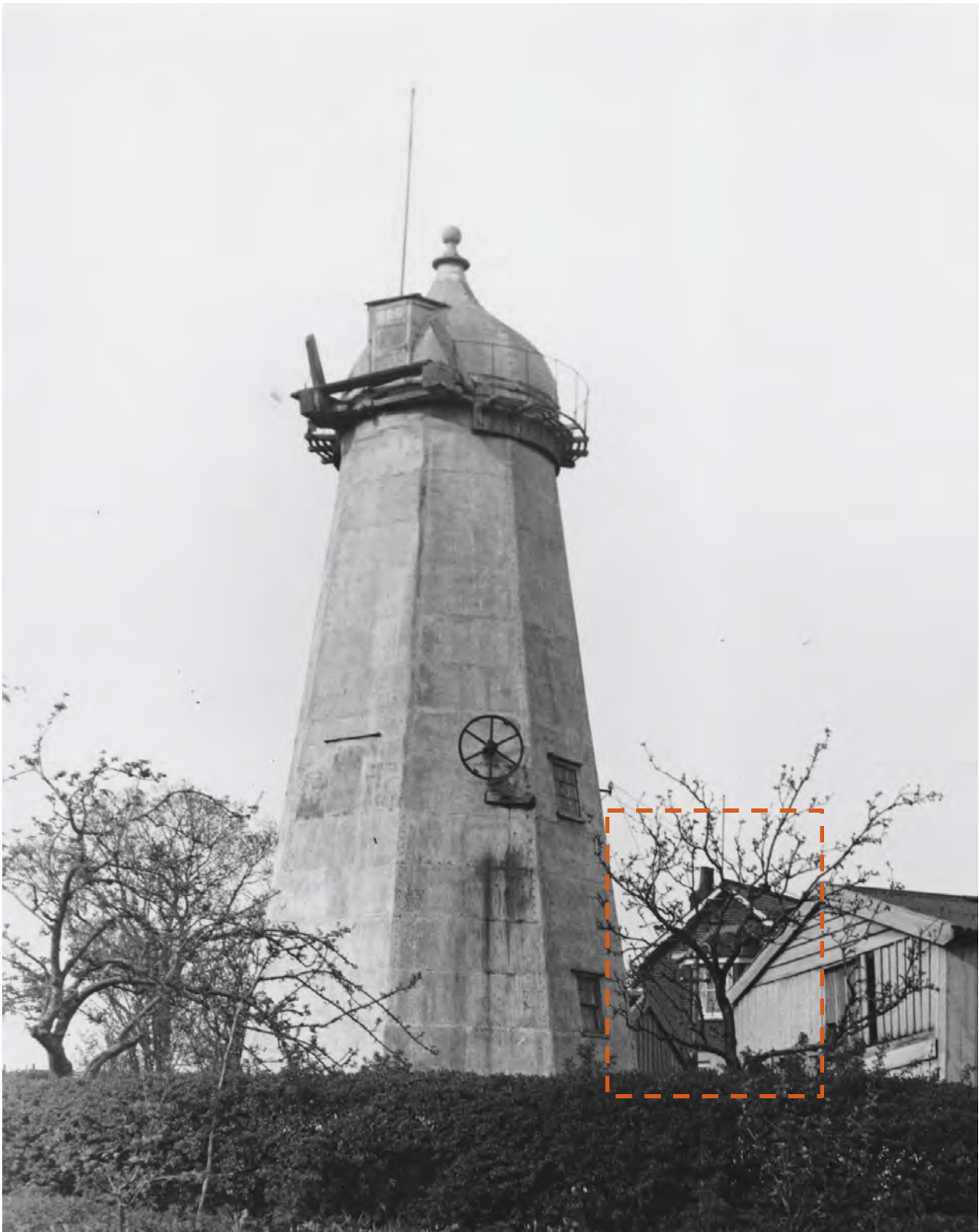
Figure 11. The image is probably from 1937. The Edwardian extension appears unpainted behind the mill ©Mills Archive
