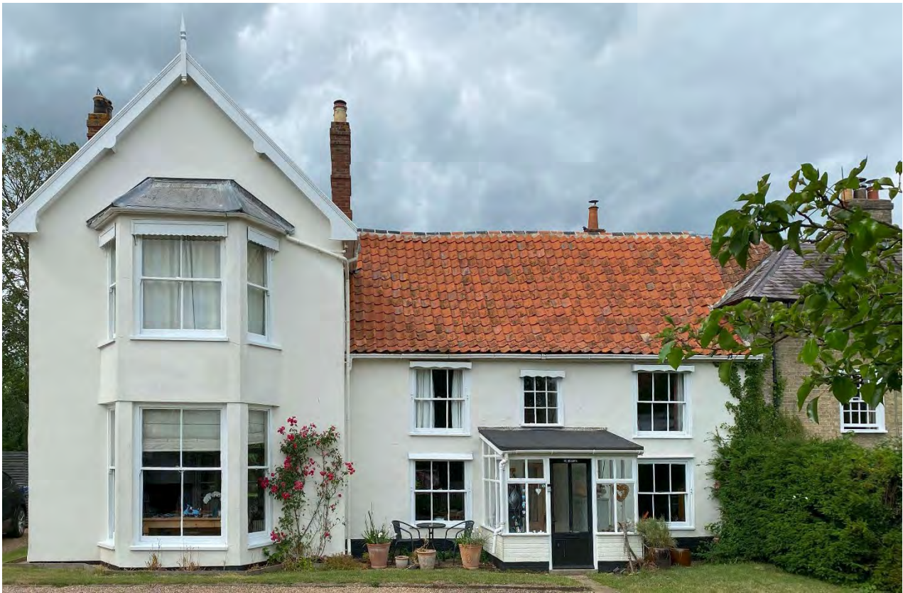
Figure 18. View of a similar extension to a cottage in Laxfields High St
