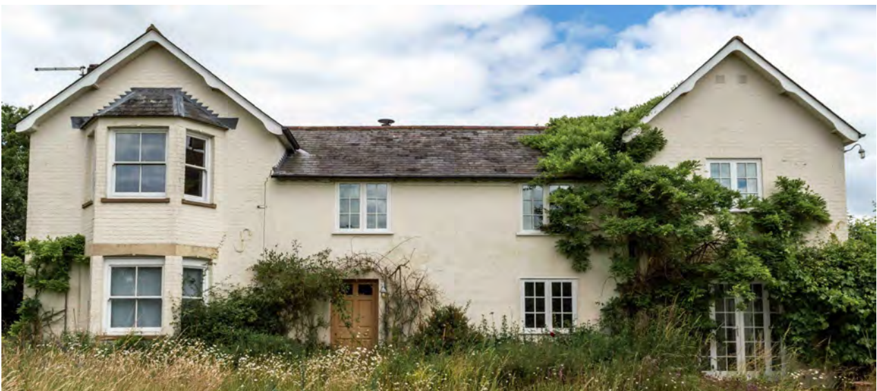
Figure 17. Despite the attempt to create a symmetrical design, the extensions vary in width and detailing.
