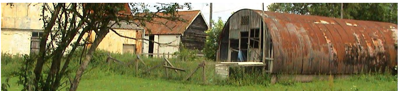
Figure 14. The 1998 auction of the house noted a Nissen structure on the grounds.
