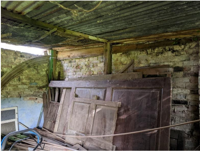
Photo 1 Internal view of shed to be demolished (i)
