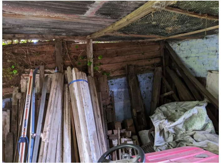
Photo 2 Internal view of shed to be demolished (ii)
