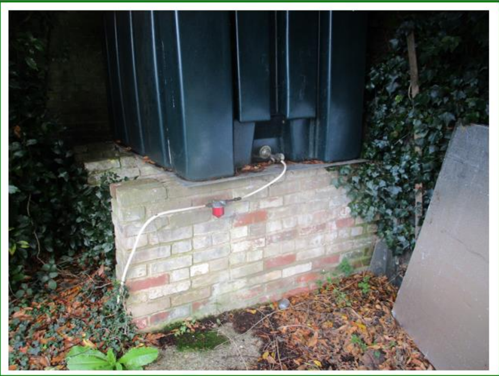
Photo No.5: Bunded fuel tank noted on western face of the outbuildings located SE of the hall itself
