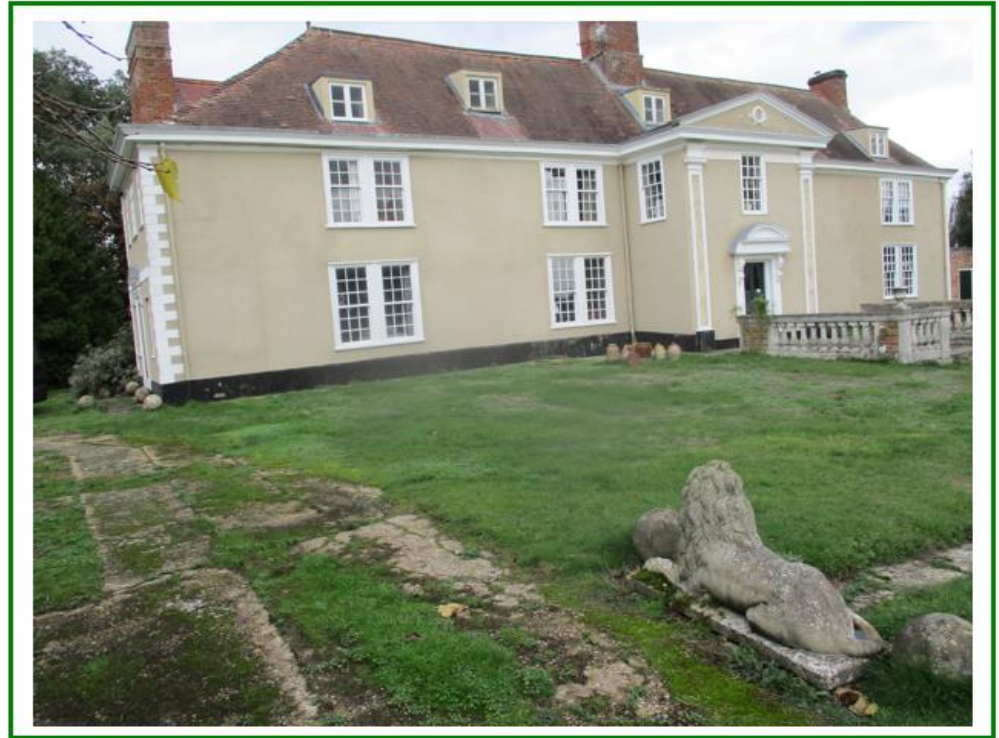
Photo No.2: Facing slightly NE from outside the SW corner of Clopton Hall showing the rear (southern) face of the building
