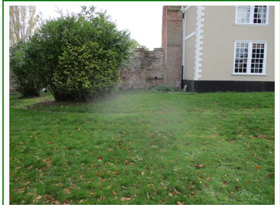
Photo No.10: Facing south from outside the NE corner of Clopton hall showing the rear of the outbuildings area
