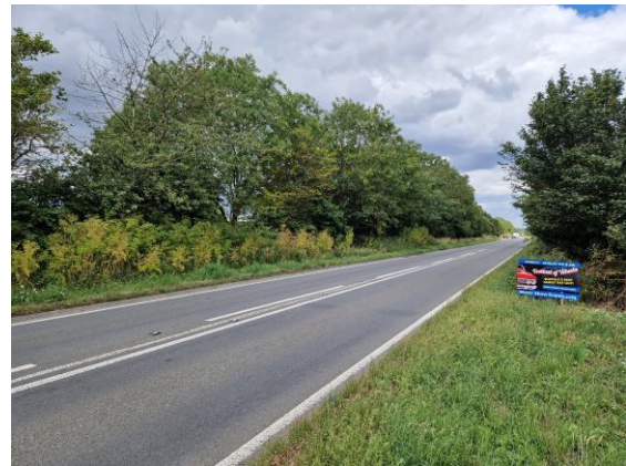
LOOKING NORTH ALONG A140 FROM THE LAY-BY GRASS VERGE OPERSITE PROPOSED NEW SITE ACCESS
