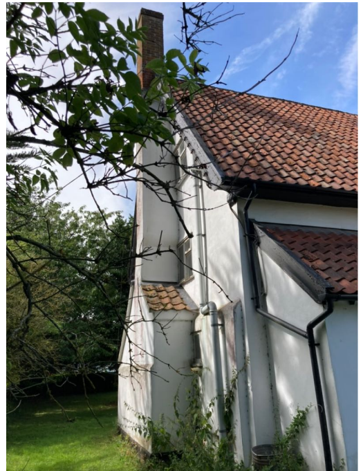
South elevation from West
