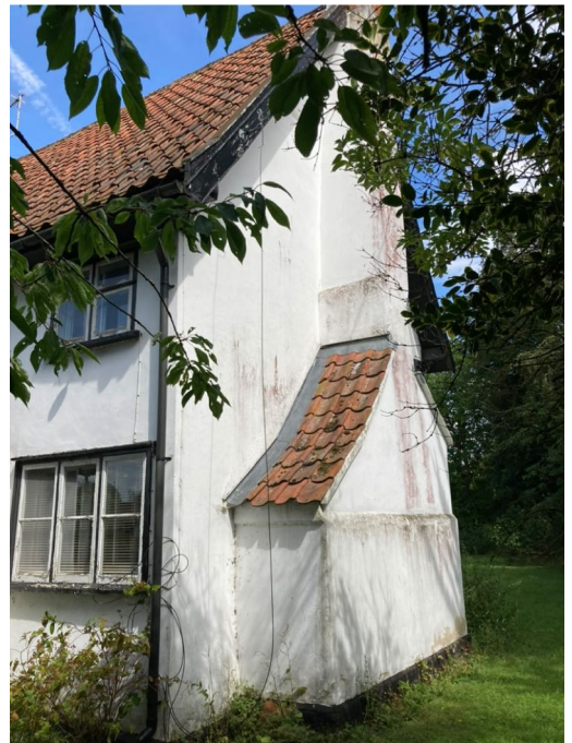
South Elevation from East
