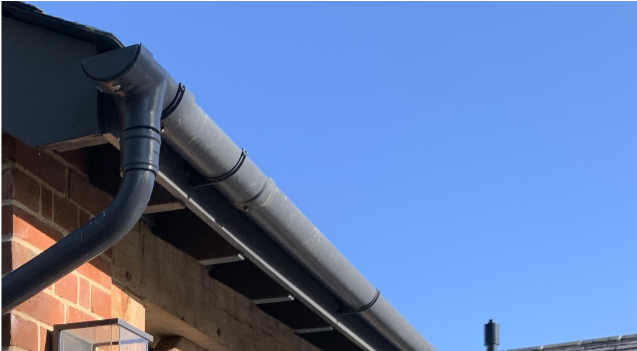
Images of existing rainwater goods.
