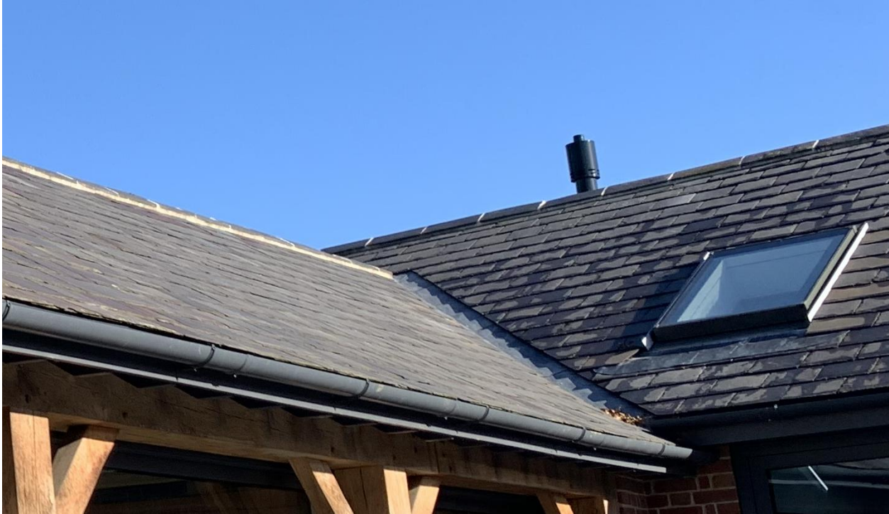
Image of existing rooflight.
