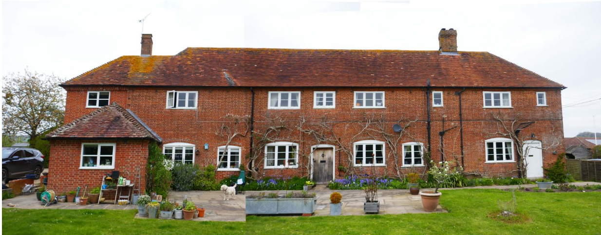
Photos of the existing building - Garden elevation
