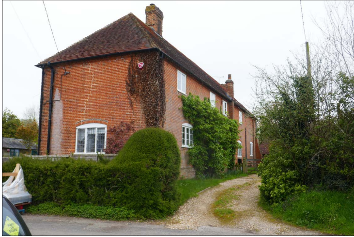
Photos of the existing building - rear elevation
