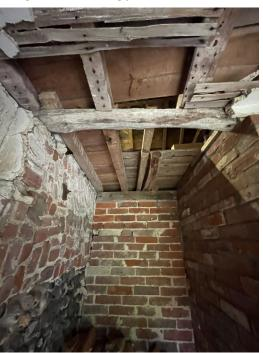
This area was chosen for the stairs specifically because the joists above the coal store have been cut and trimmed in the past, indeed we believe it is possible this area may have included a loft ladder for internal access to the space. The masonry in this area should not need altering as the winding stair sits entirely within the existing void.
