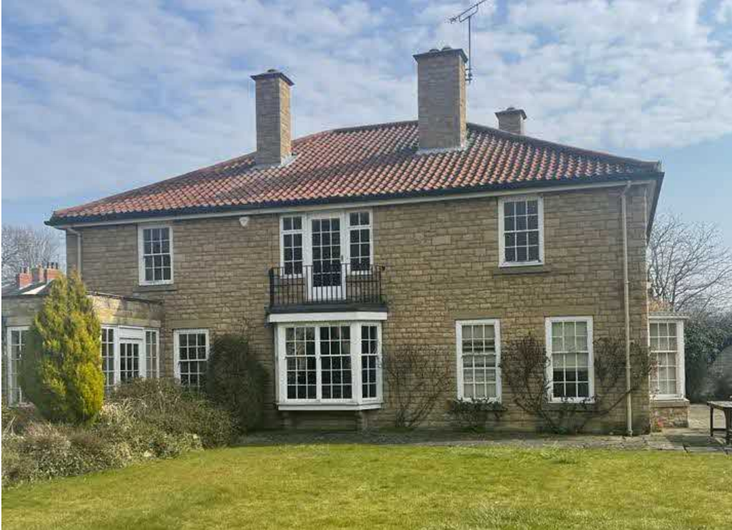
West elevation of host building, showing stone walls and pantiled roof
