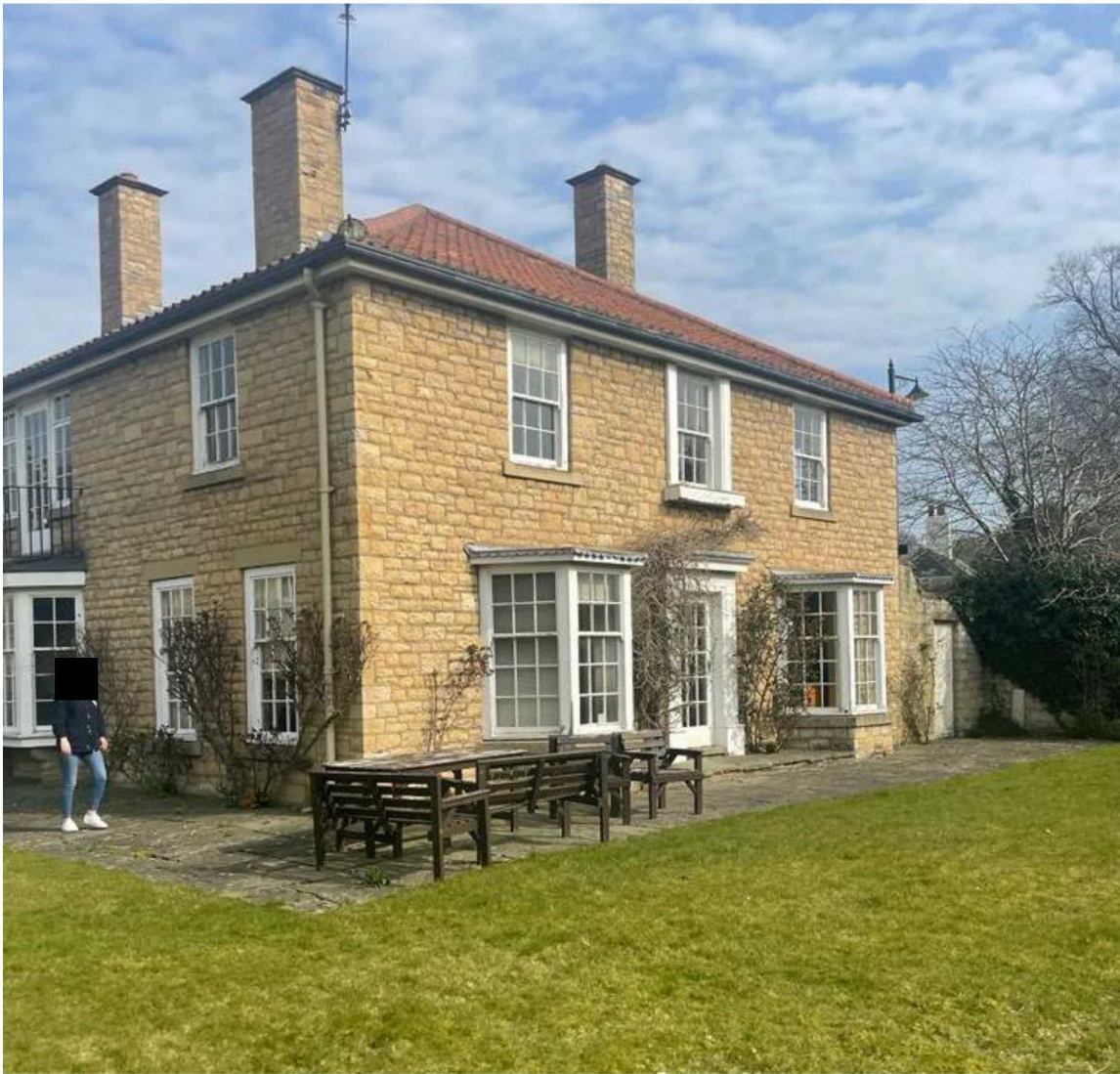
South elevation of host building, showing projecting bay windows
