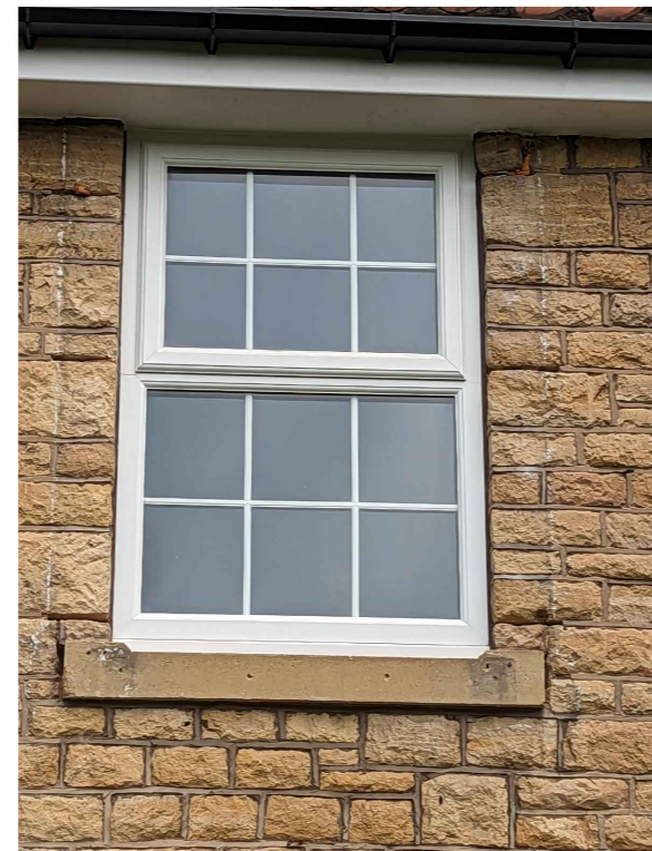
First Floor Office
