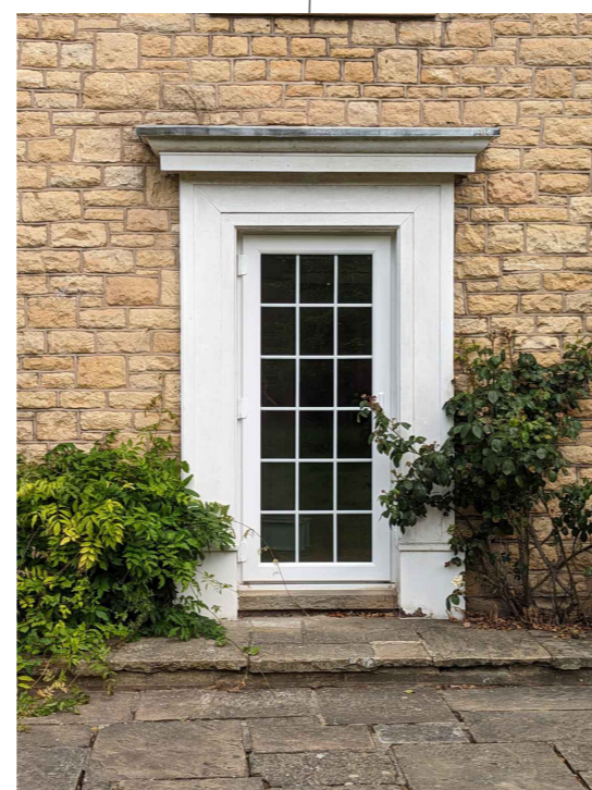
Ground Floor Office Personnel Access
