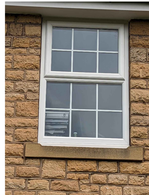
First Floor Office
