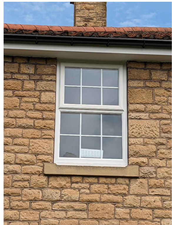
First Floor Office
