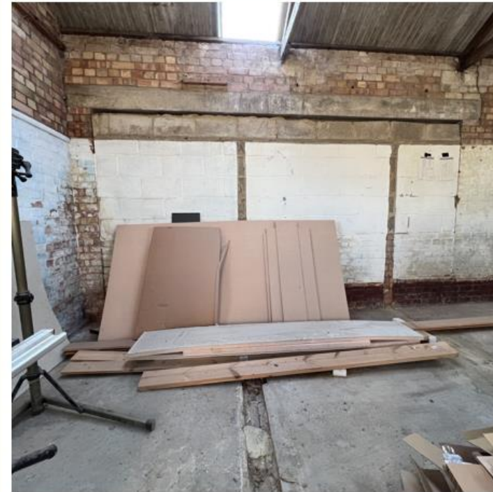
Photo No.16: Taken facing south of the workshop area timber storage
