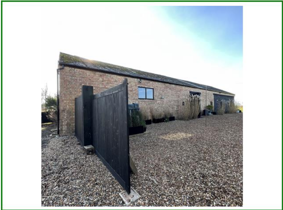
Photo No.2: Facing SW from the NE corner of site showing the gravelled parking area north of the site building
