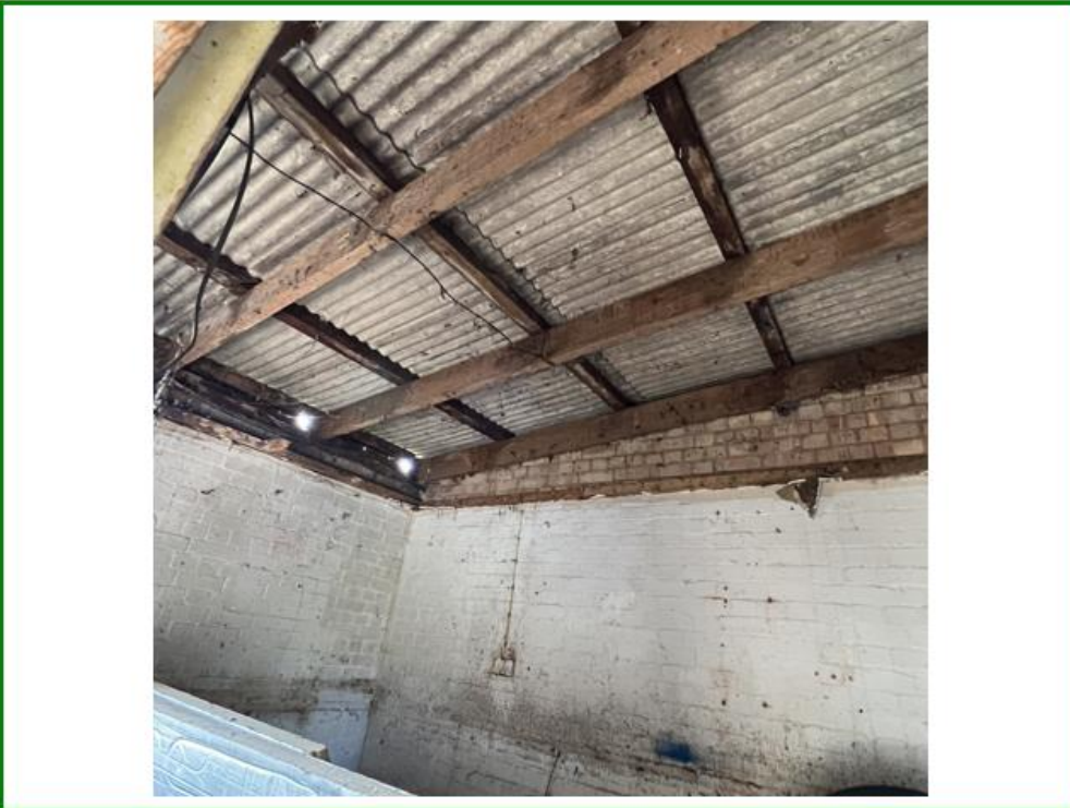
Photo No.10: Showing potentially asbestos roofing beneath newly installed corrugated metal roofing atop stables
