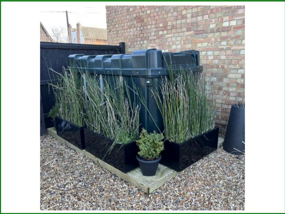
Photo No.3: Bunded oil storage on NE corner of the building and atop a concrete base – visual or olfactory evidence of spillages
