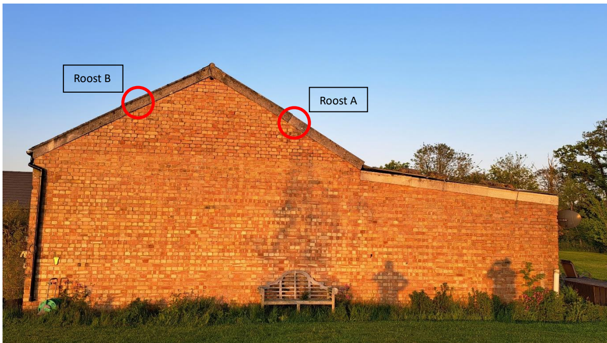
Figure 2 Emergence locations from combined surveys – west elevation. Roost A (Survey 1 and 2), Roost B (Survey 2 and 3)
