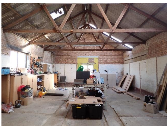
Light internal areas of the barn
