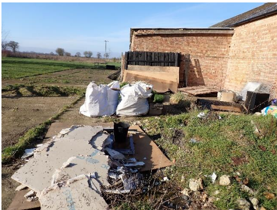
Piles of building materials, vegetation, and spoil
