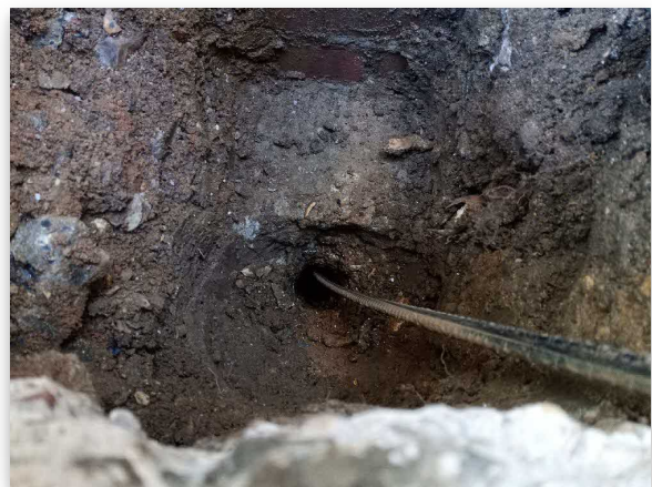
Fig 1.2: Trial Hole 1 Footing
