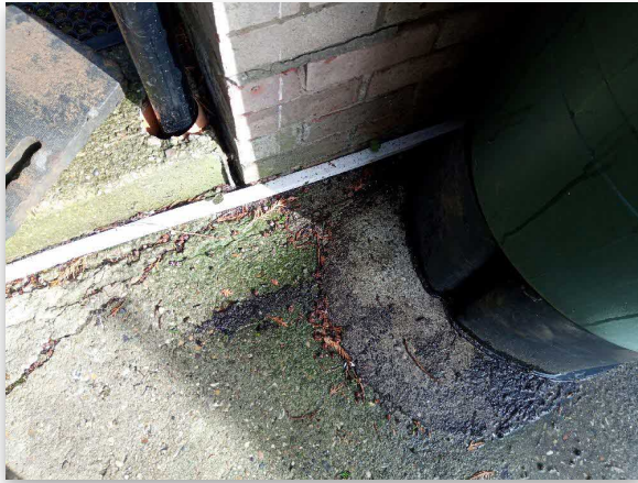
Fig 2.1: Trial Hole 2 Location
