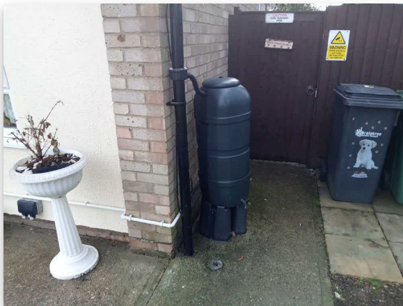
Fig 4.1: RWP1 area of excavation
