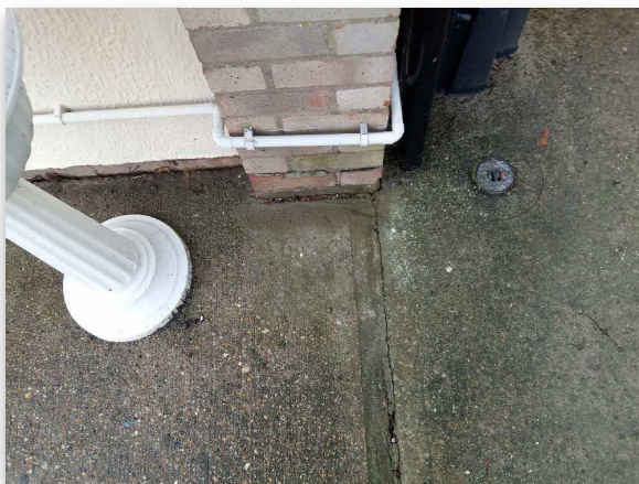
Fig 1.1: Trial Hole 1 Location
