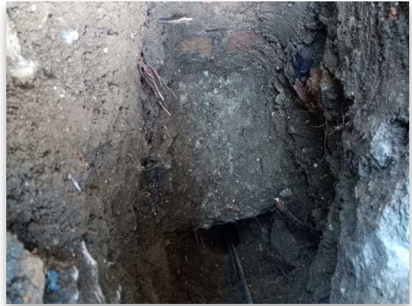
Fig 2.2: Trial Hole 2 Footing
