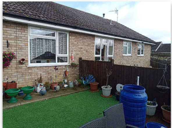
Fig 4.2: Rear of the property
