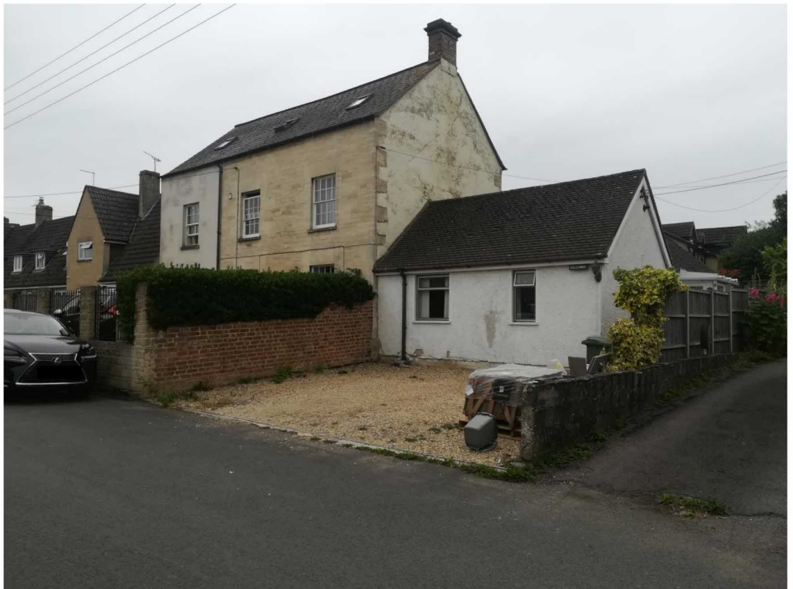
Sholom shown to the east with Sholom Cottages beyond
