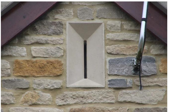
4. Air slit and barge board
