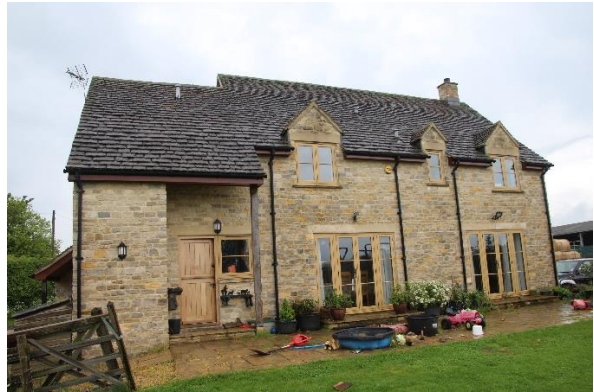
2. House from the north
