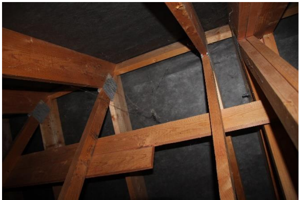
5. Loft space with membrane and webs
