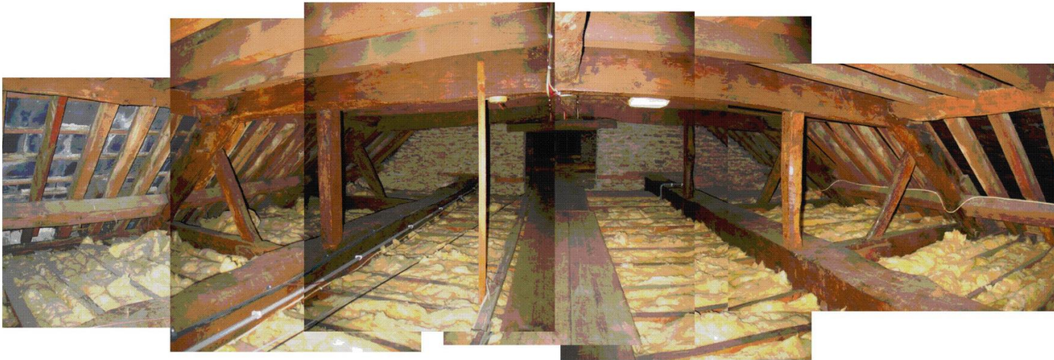
Composite view of Truss No. 6 from the north
