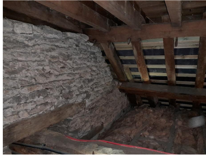
Close up on view to side of wall showing roof slope with modern battens.
