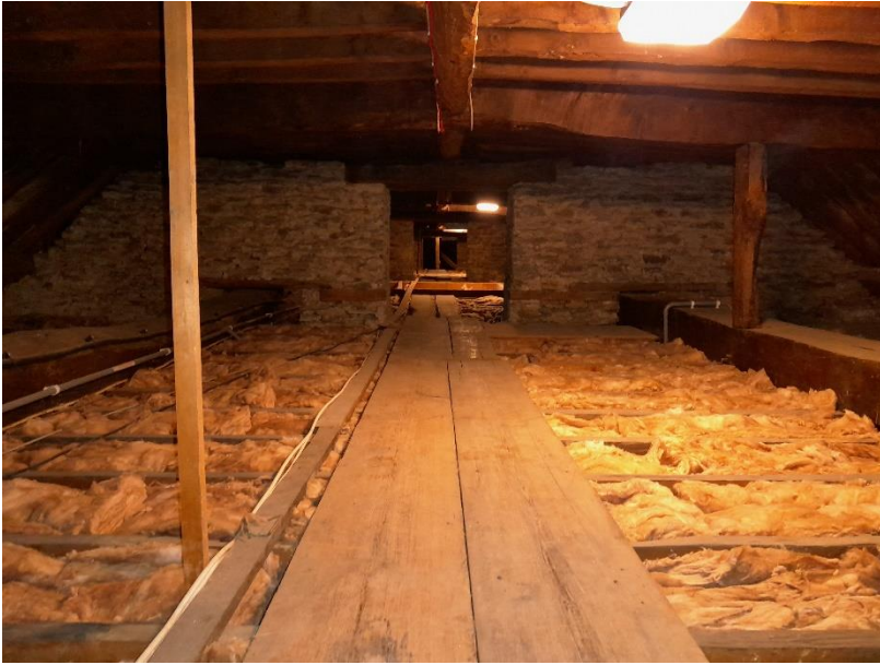
View north of wall to which fire stopping alterations are proposed.
