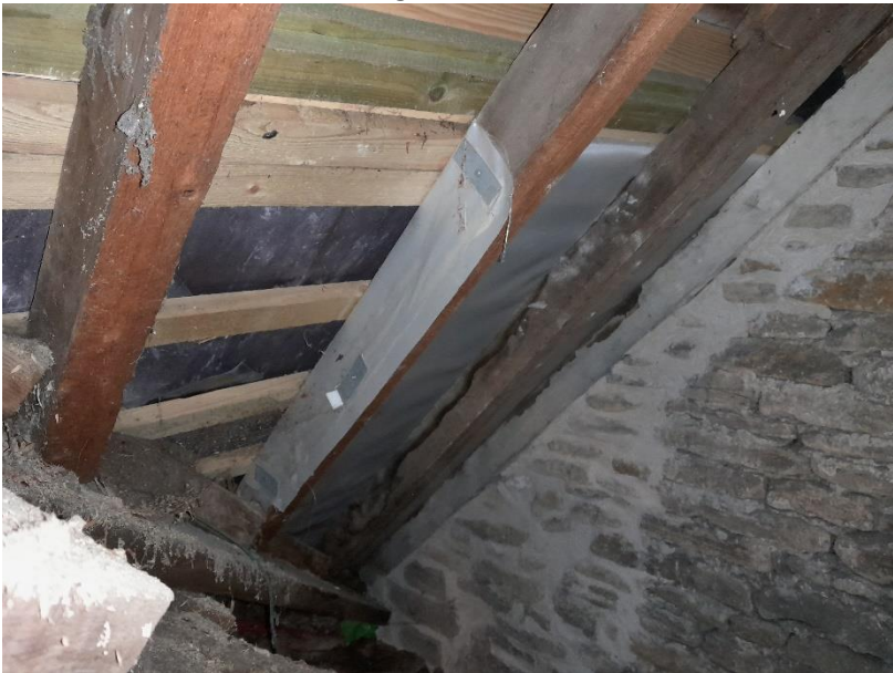
View along top of wall head demonstrating gap between wall head and underside of roof coverings.
