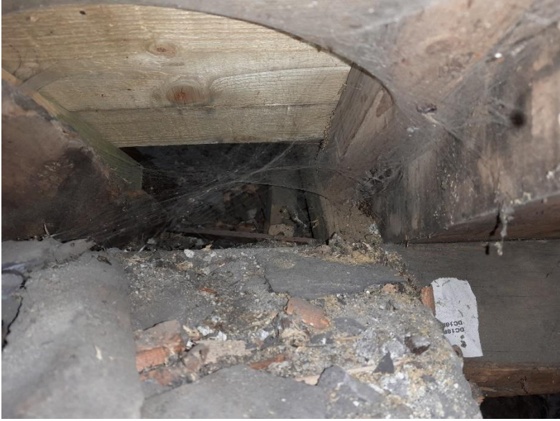
View along top of wall head demonstrating gap between wall head and underside of roof coverings.
