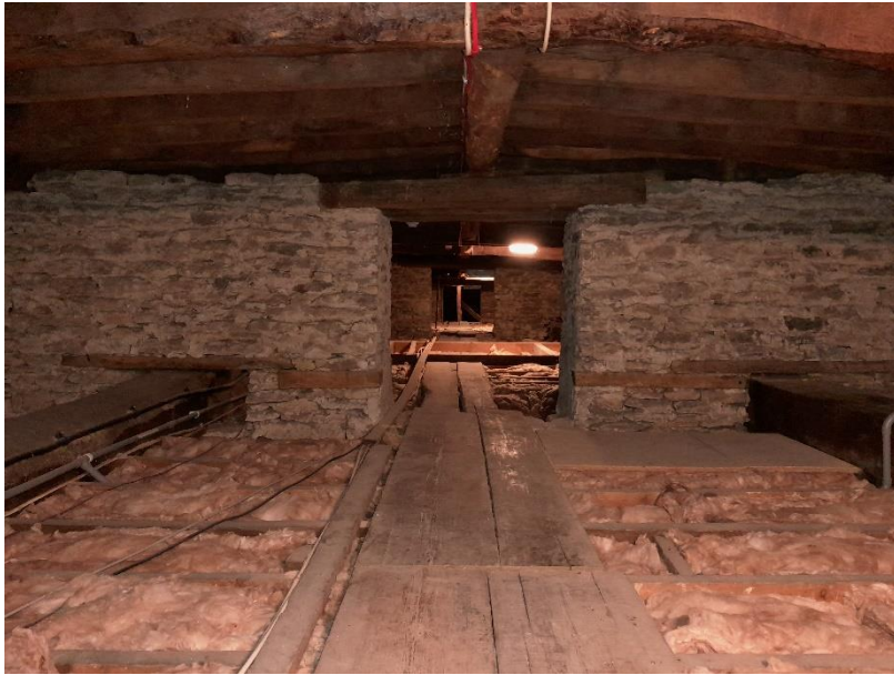
View of other side of proposed compartmentation wall from previous photos.
