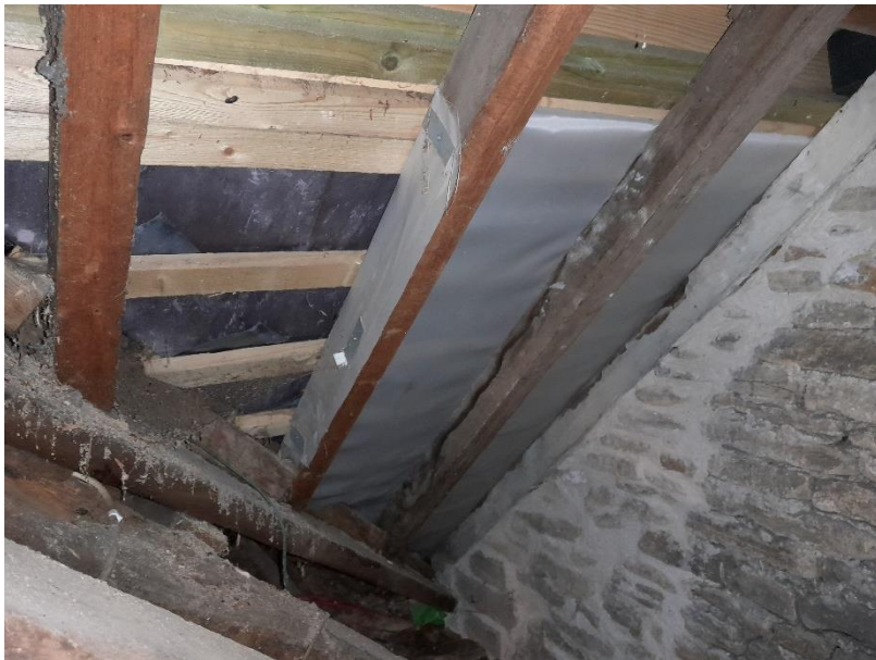
Example of existing fire stopping installed to different sections of roof
