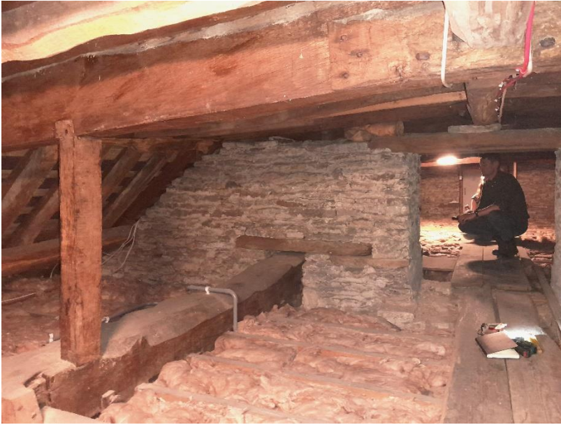
View of section of wall to receive fire stopping alterations
