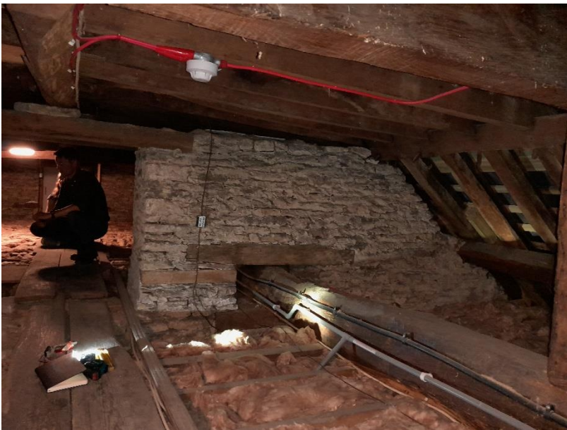
View of section of wall to receive fire stopping alterations
