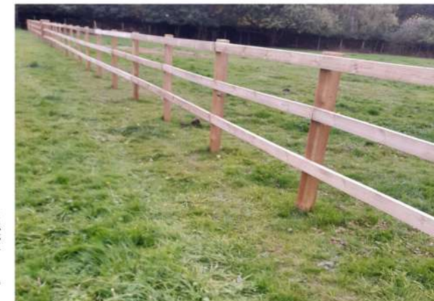
Photo B 3 bar post and rail fence 1.2m high
