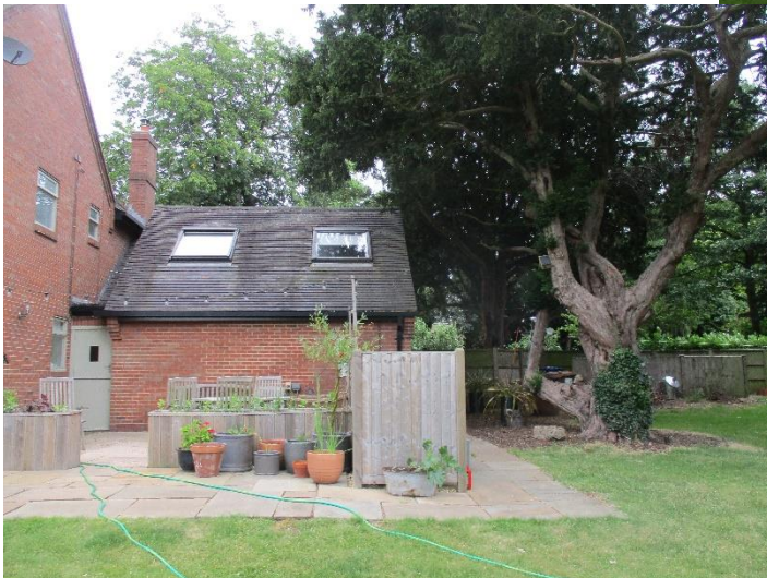
Photo Three – Showing T10 and area of proposed extension
