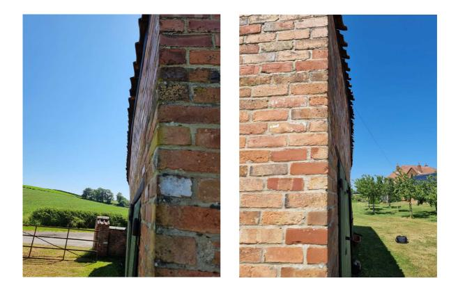
The building in its current state could be considered as detrimental to local visual amenity, furthermore it is considered that unless the roof is removed and the top 1m of the walls are re-built the building is in danger of collapse. This raises significant safety concerns for my client and the wider public given the proximity of the public highway. Undertaking the proposed roof works would preserve and enhance the building as part of the existing landscape in accordance with the NPPF.
