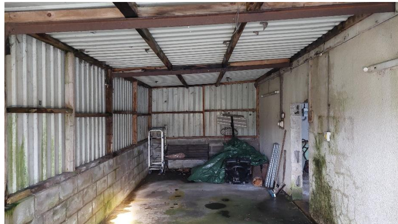
Photograph 31: Interior of the milking shed.
