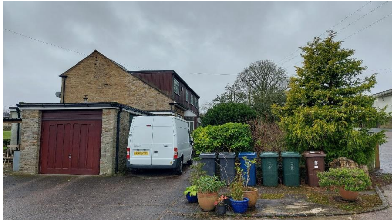
Photograph 7: Northern gable end of the existing farmhouse.
