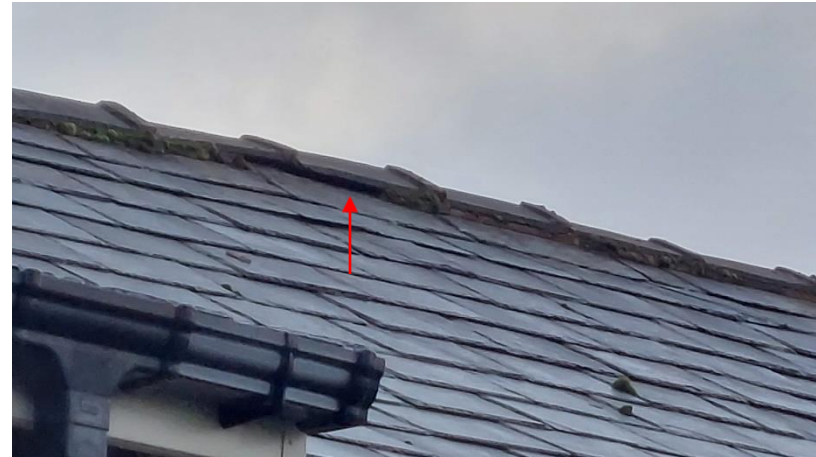
Photograph 26: Red arrow indicates potential ingress/egress for bats. The feature here is the right most arrow in Photograph 25.
