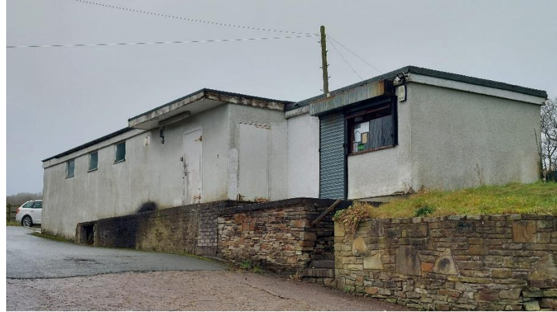
Photograph 9: Eastern aspect of the former milking shed.
