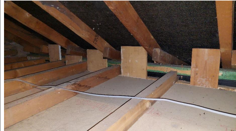
Photograph 14: Floor of Loft 1.
