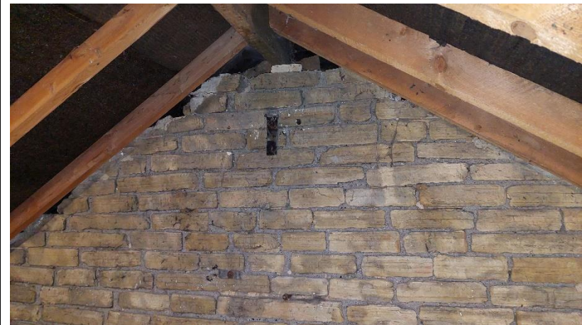
Photograph 12: Gritstone brick party wall of Loft 1.
