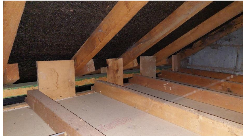
Photograph 13: Floor of Loft 1.
