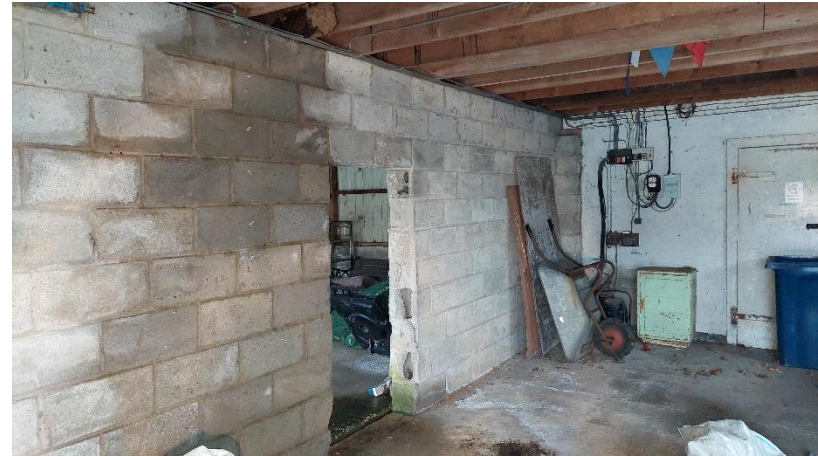
Photograph 30: Interior of the milking shed.
