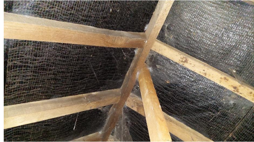
Photograph 18: Roof structure of Loft 2.
