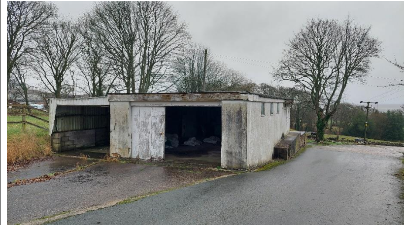
Photograph 10: Southern aspect of the former milking shed.
