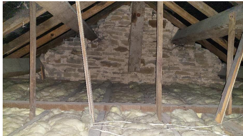
Photograph 15: Party wall and woollen loft insulation of Loft 2.
