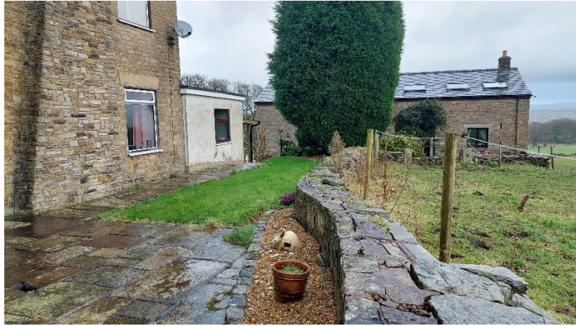
Photograph 5: Garden to the rear (east) of the existing farmhouse.
