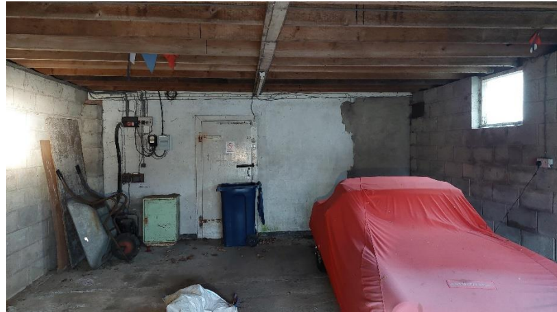
Photograph 29: Interior of the milking shed.
