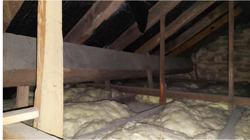
Photograph 17: Floor and wooden rafters, uprights and supporting beams of Loft 2.
