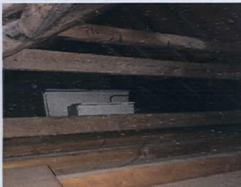
Figure 7: House roof void
