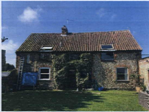
Figure 1: Eastern aspect of house
