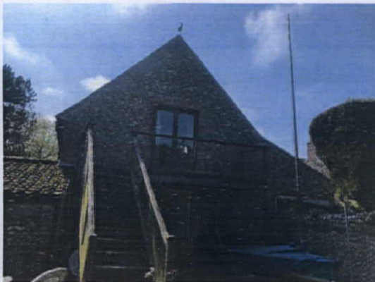
Figure 5: Northern aspect of house
