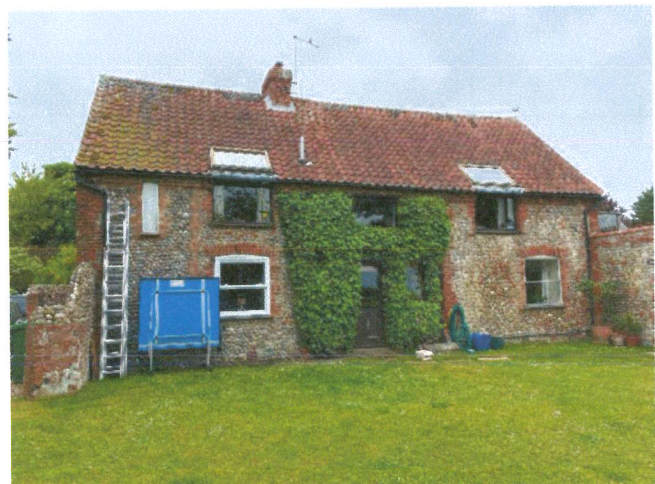
Fig. 2. View of the rear of the property
