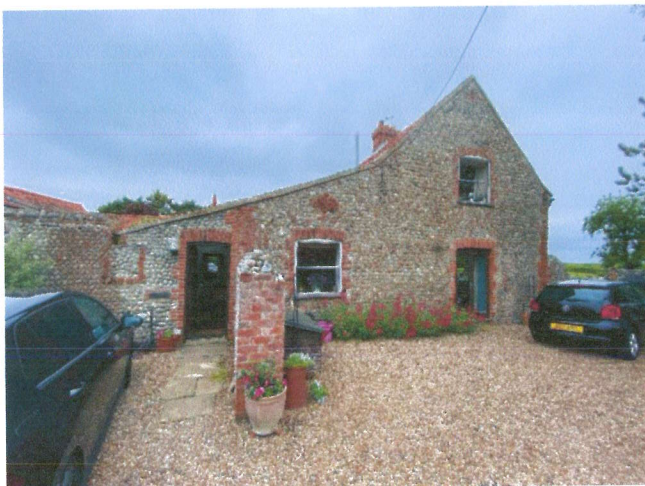
Fig. 1. View of the front/side of the property
