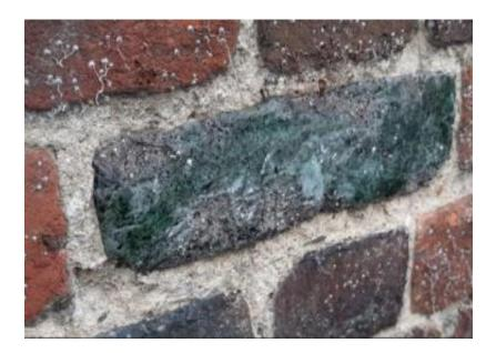
No new rendering is proposed other than to rake out cracks and hollow sheer areas of cementious render and fine fill to prevent any rainwater wash gaining access into the underlying modern walls.
