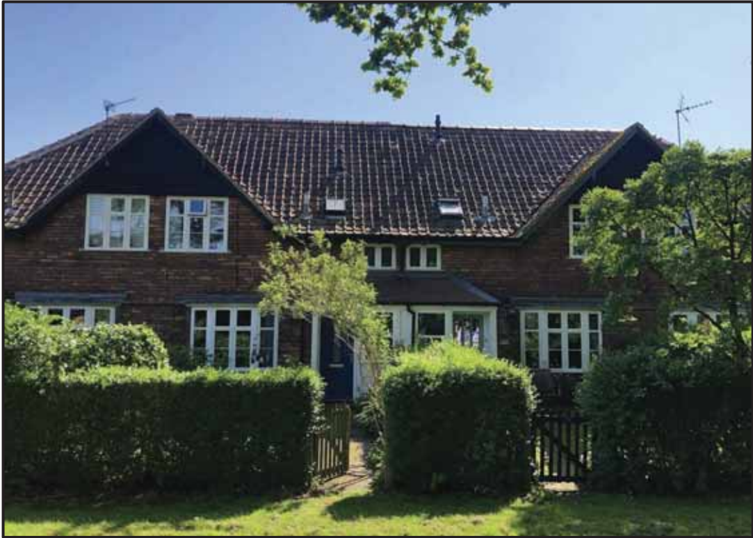
Plate 59: 5-8 Hawthorn Terrace, front elevation
