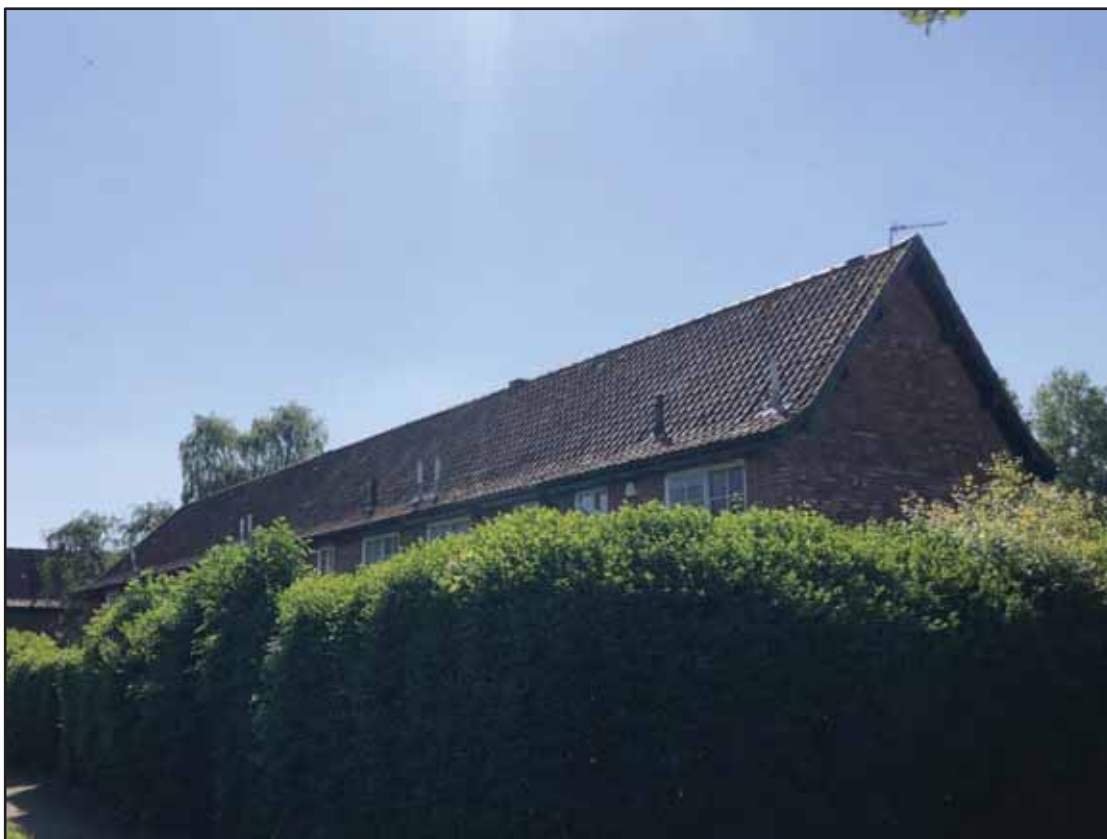
Plate 66: 1-5 Ivy Place, rear elevation
