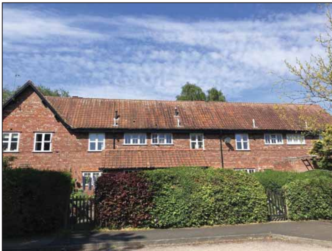
Plate 73: 16-20 Ivy Place, rear elevation
