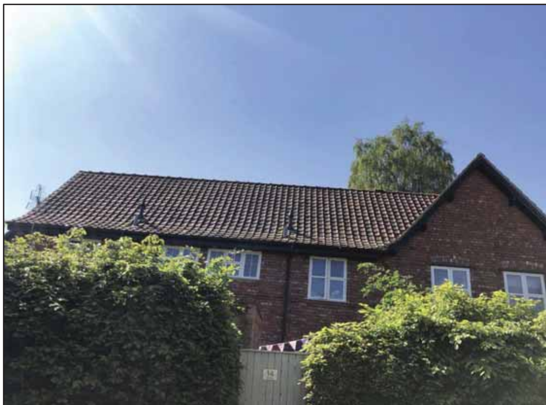
Plate 70: 13-15 Ivy Place, rear elevation
