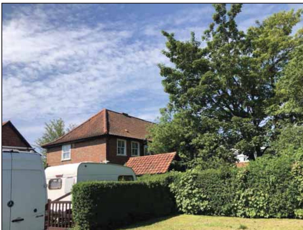
Plate 2: 14-18 Sycamore Place, rear elevation
