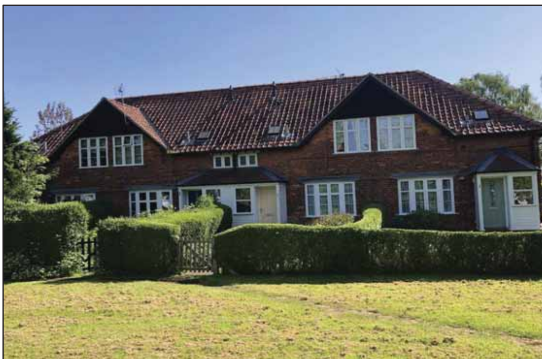
Plate 57: 1-4 Hawthorn Terrace, front elevation
