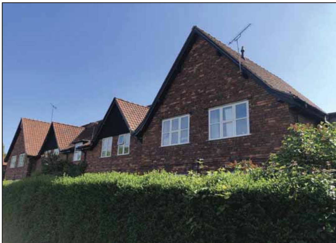
Plate 61: 9-12 Hawthorn Terrace, front elevation
