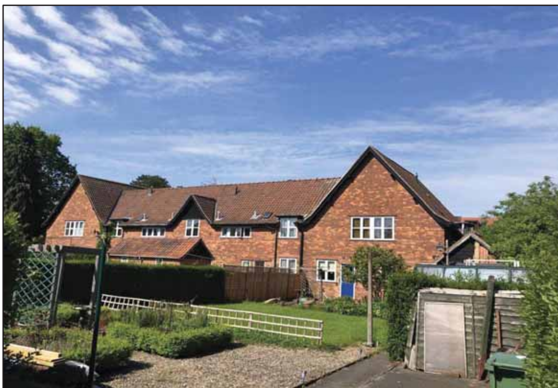
Plate 64: 9-12 Hawthorn Terrace, rear elevation
