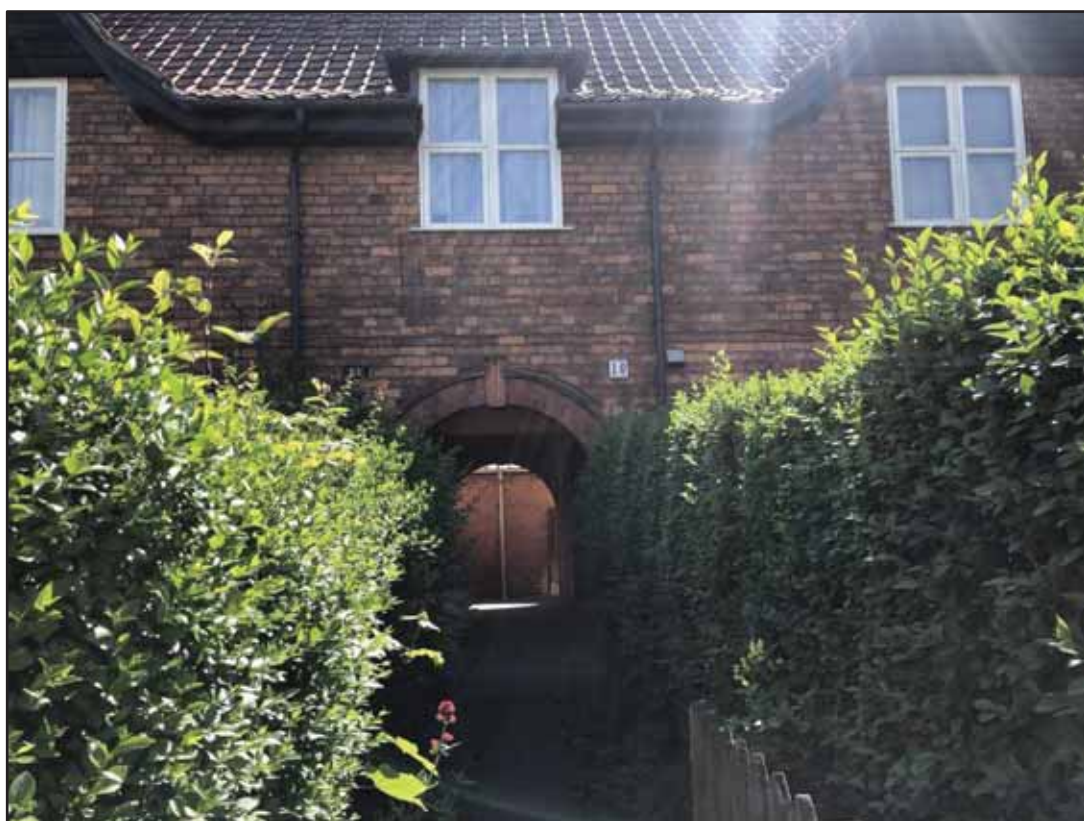
Plate 62: 9-12 Hawthorn Terrace, front elevation
