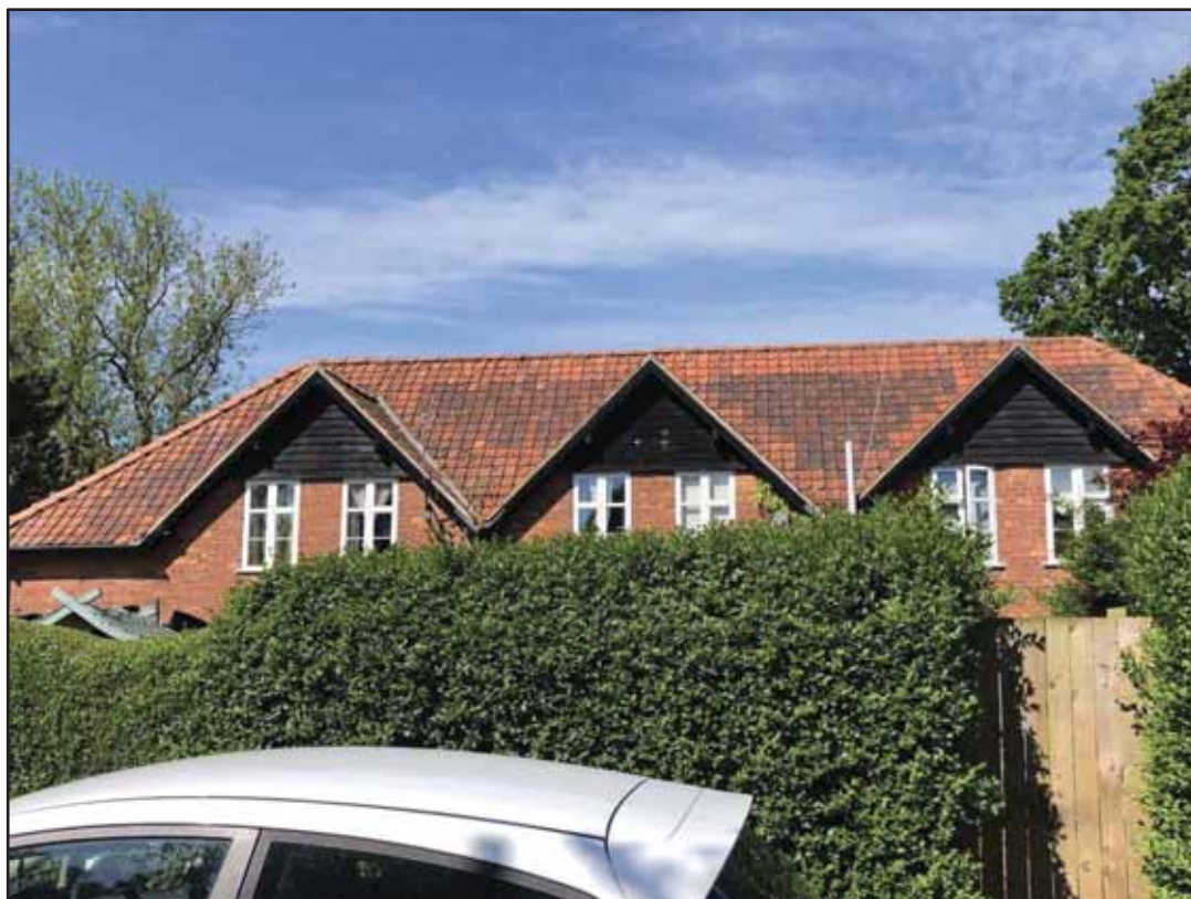
Plate 58: 1-4 Hawthorn Terrace, rear elevation
