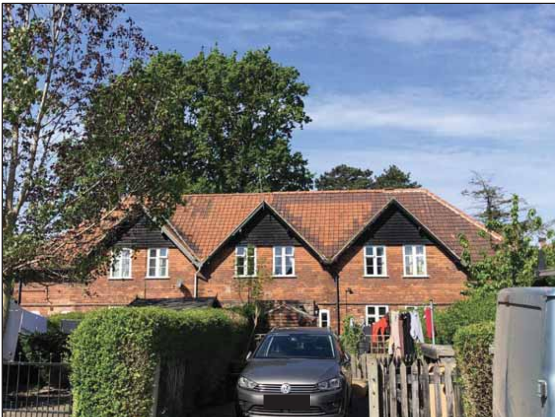
Plate 60: 5-8 Hawthorn Terrace, rear elevation
