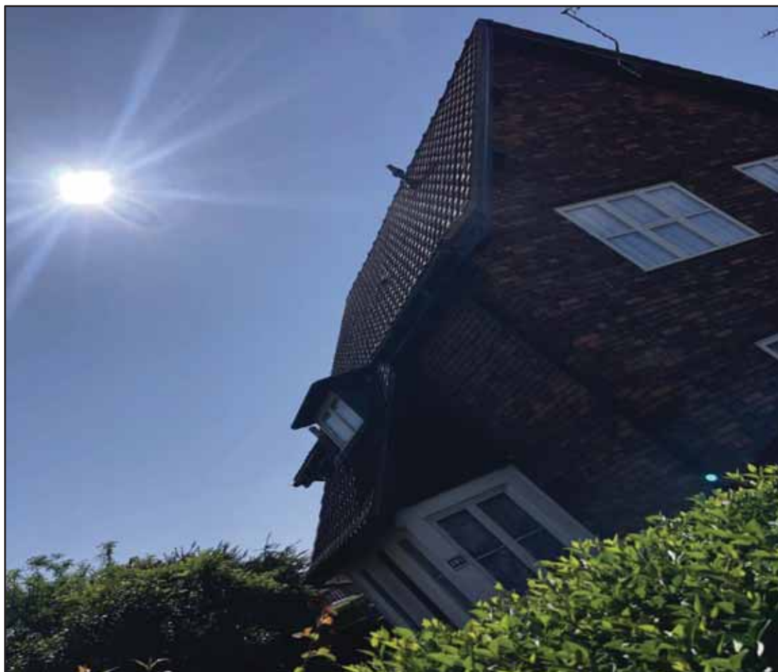
Plate 63: 12 Hawthorn Terrace, side elevation
