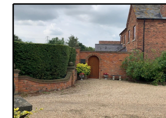
C - VIEW FROM THE ENTRANCE TO THE DRIVE OF MILL PADDOCKS WITH ON THE ROOF EXTENSION VISIBLE
