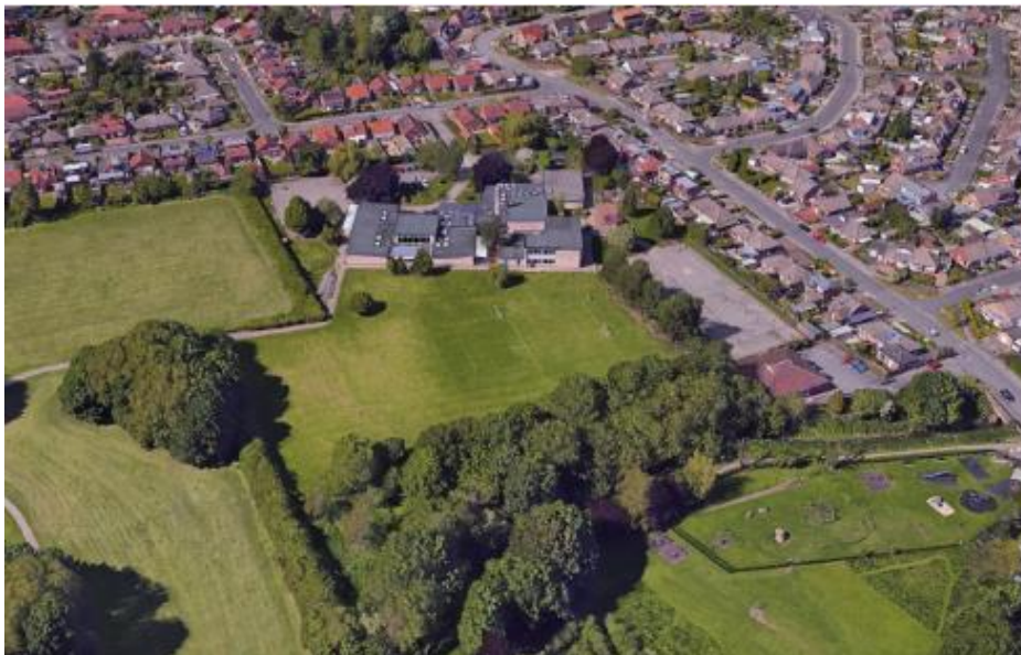
Figure 1 – Aerial image of site
